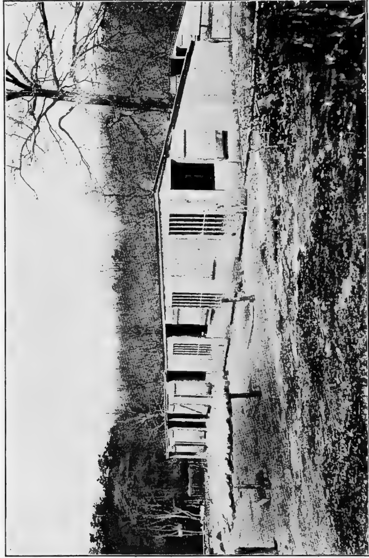
FIG. 18. A good house for breeding ducks. It is 20 feet deep, 40 feet long, 7 feet high in front and 4 feet in the rear and will accommodate 200 breeders. ( Photograph from the Bureau of Animal Industry, U. S. Department of Agriculture. )
