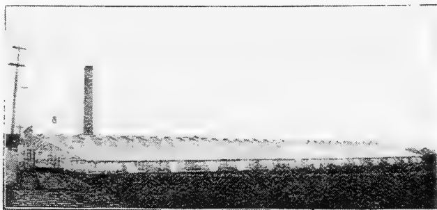
D. L. TAPPAN'S VEGETABLE FORCING HOUSE, AT ARLINGTON, MASSACHUSETTS.
