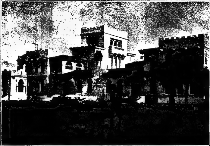
MRS. KING'S NEW FIREPROOF RESIDENCE, UNDER CONSTRUCTION AT SANTA GERTRUDIS.
