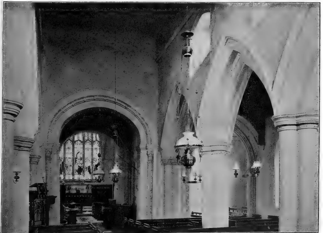
ANSTEY CHURCH : THE NAVE LOOKING EAST
