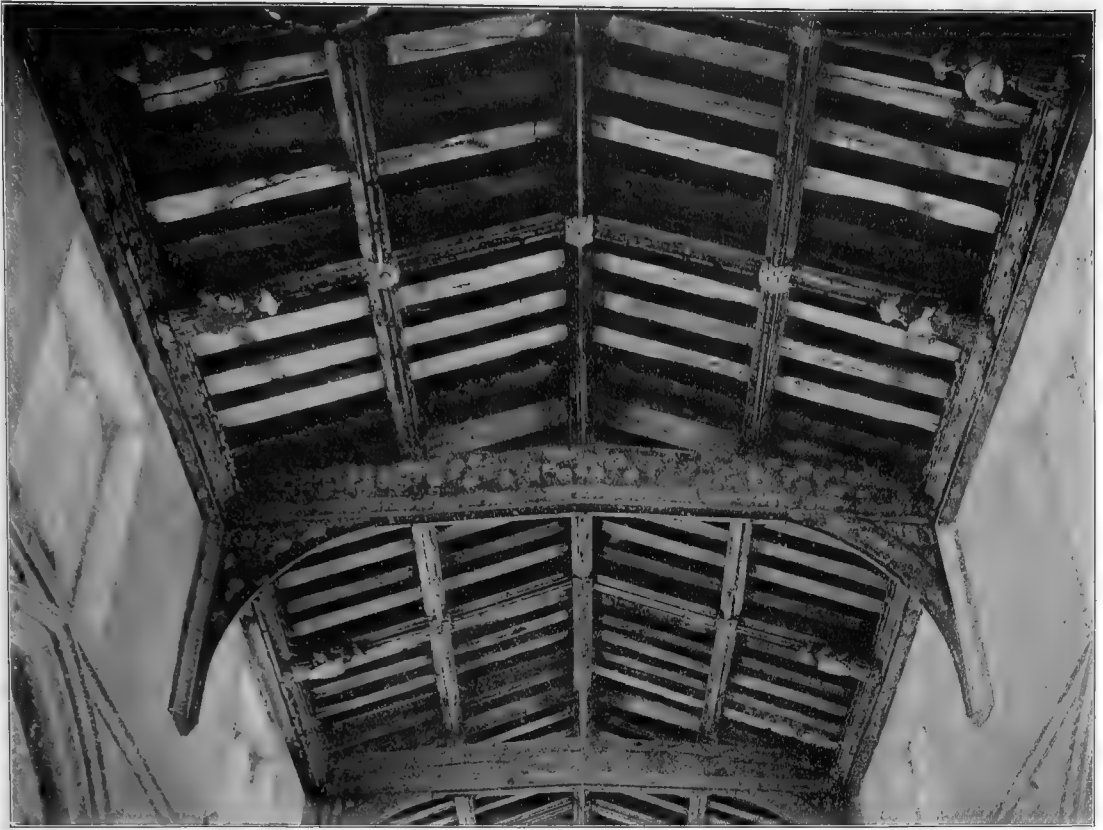
FURNEUX PELHAM CHURCH : THE NAVE ROOF
