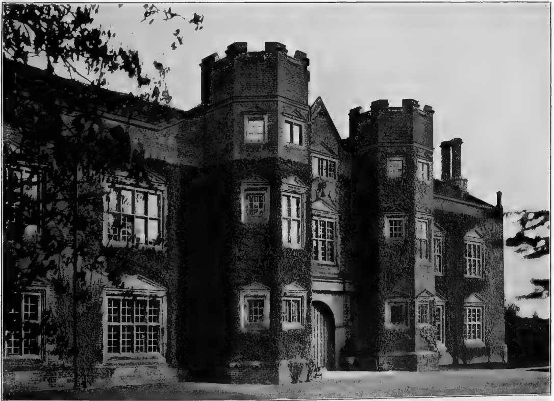
HADHAM HALL : PRINCIPAL FRONT
