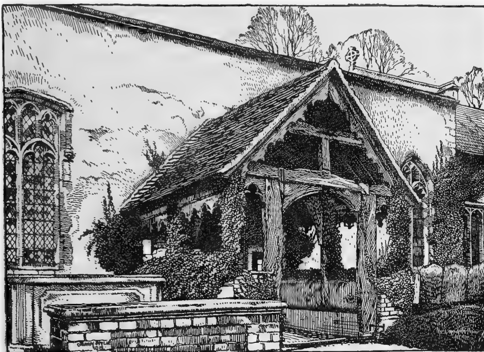
CHURCH PORCH, LITTLE HADHAM
