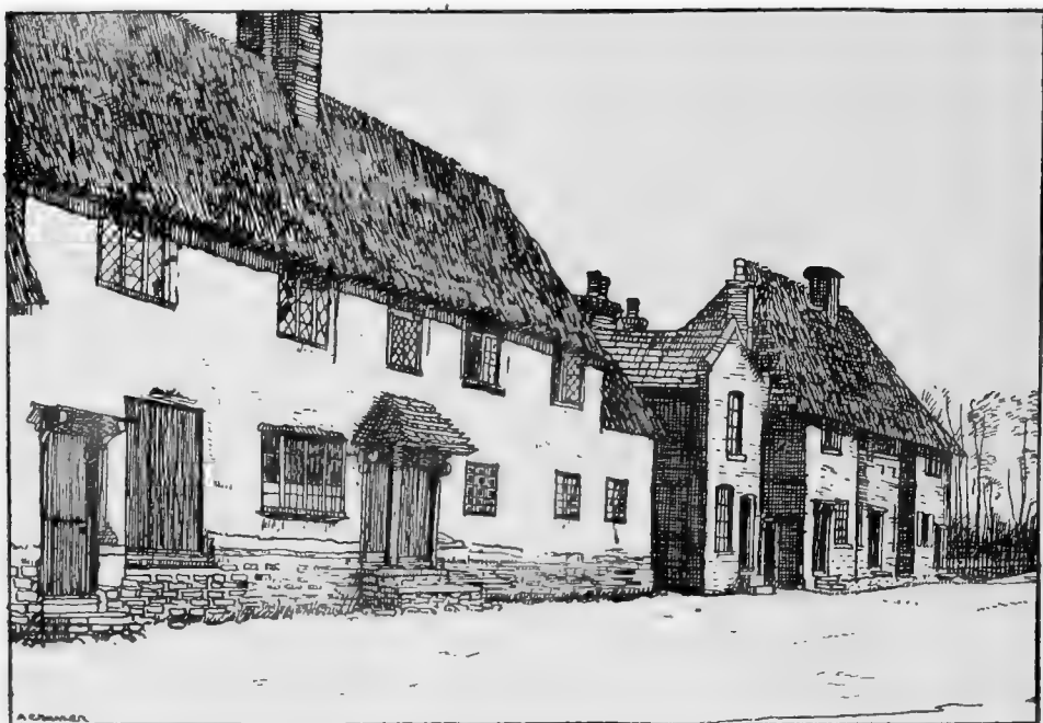
SOUTH END OF MAIN STREET, BARKWAY
