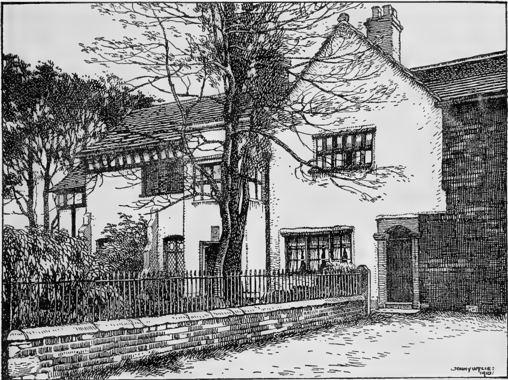
HYDE HALL : ENTRANCE FRONT
