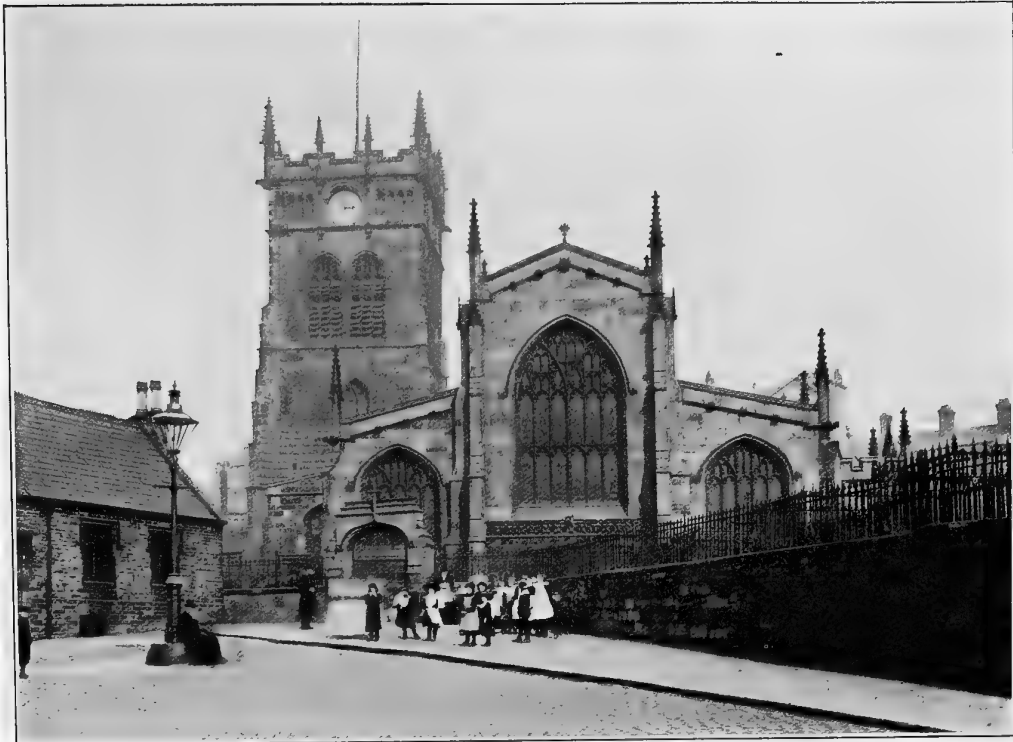
WIGAN CHURCH, FROM THE NORTH-WEST, SHOWING TOWER
