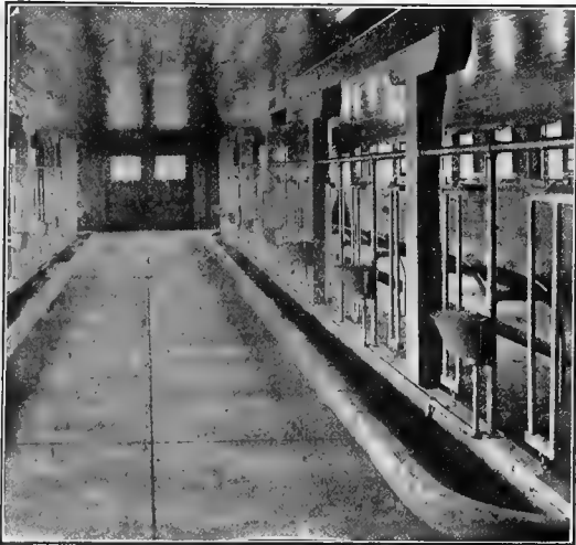
FIG. 73.—INTERIOR VIEW OF DAIRY BARN, SHOWING FEEDING ALLEY, MANAGERS, AND INDIVIDUAL WATERING DEVICE. Bowen & Quick, Auburn, N. Y.
