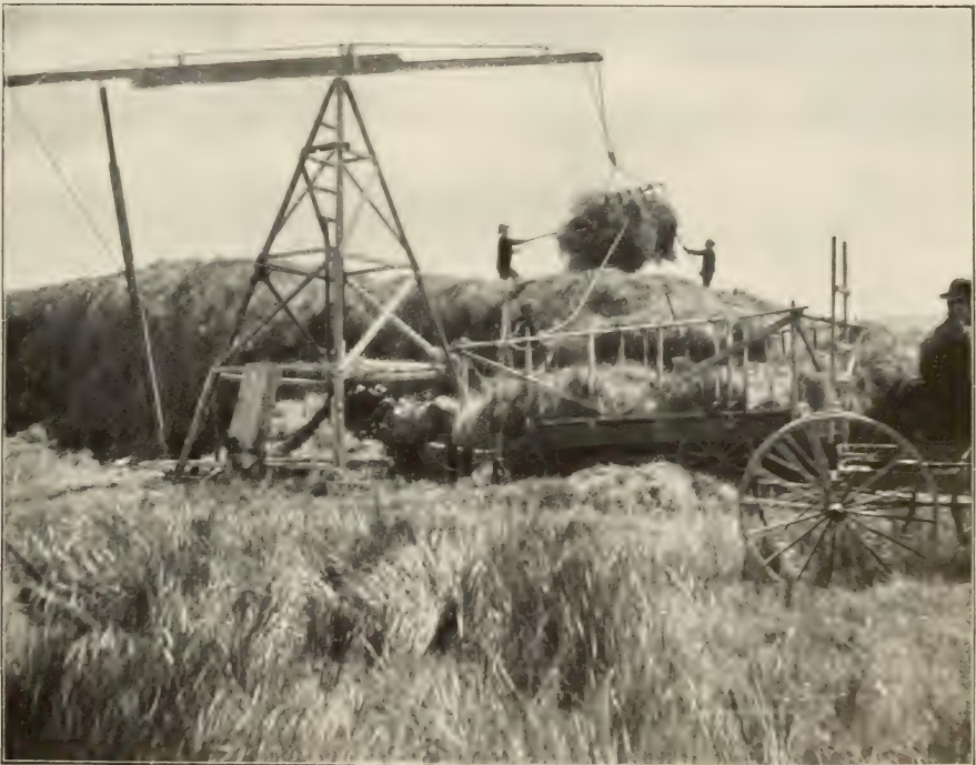
FIG. 2.—DERRICK STACKER, SHOWING DETAILS.
