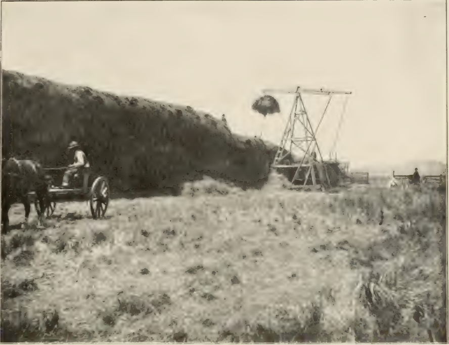
FIG. 1.—DERRICK STACKER, WITH JACKSON FORK.
