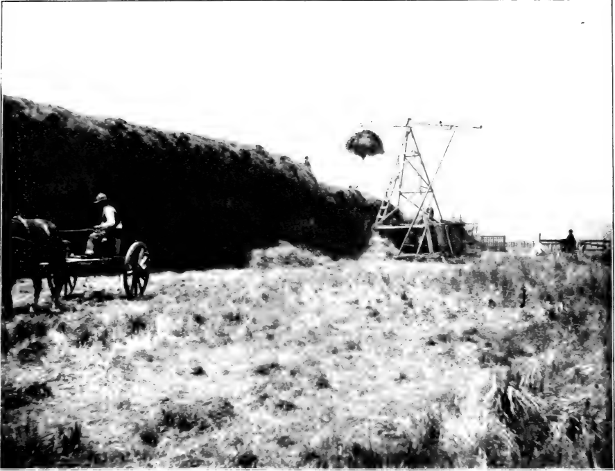
FIG. 1.—DERRICK STACKER, WITH JACKSON FORK.
