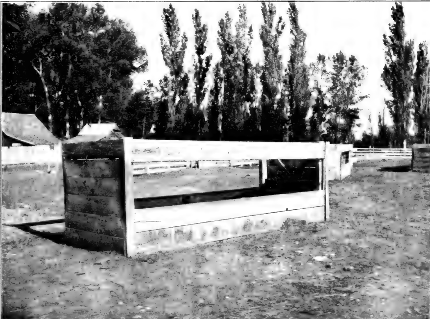
FIG. 2.—BOX RACK FOR FEEDING ALFALFA TO CATTLE.
