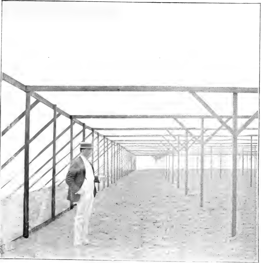
FIG. 1.—PART OF A 10-ACRE TOBACCO FIELD COVERED WITH CHEESE CLOTH, SHOWING THE DETAILS OF THE OUTSIDE STRUCTURE OF THE FRAME.
