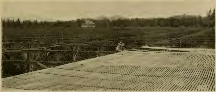
Roofing over an orange grove at the Everest Rancho, Arlington Place, Riverside County.
