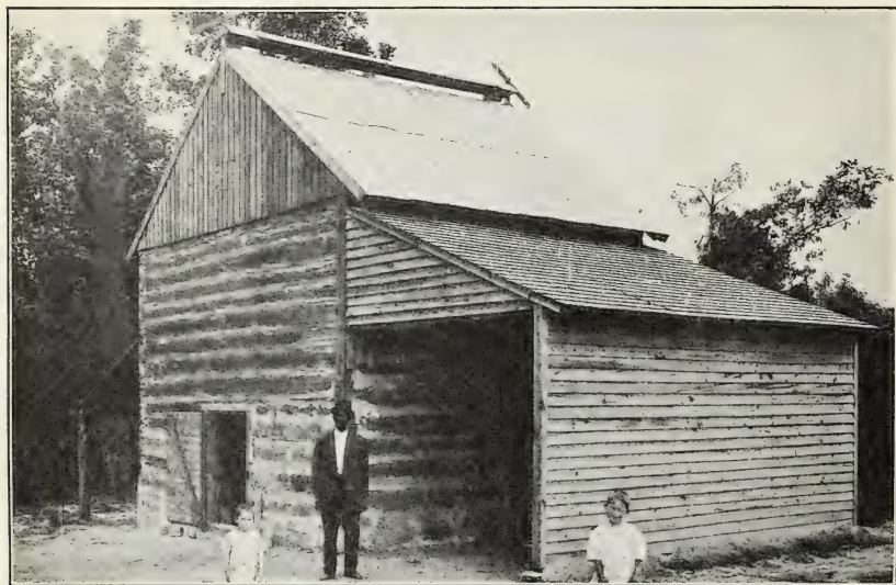
FIG. 11.—A good type of flue-curing tobacco barn, showing the ridgepole ventilator raised. The mouth of one of the bottom air inlets is seen just under the open door.
