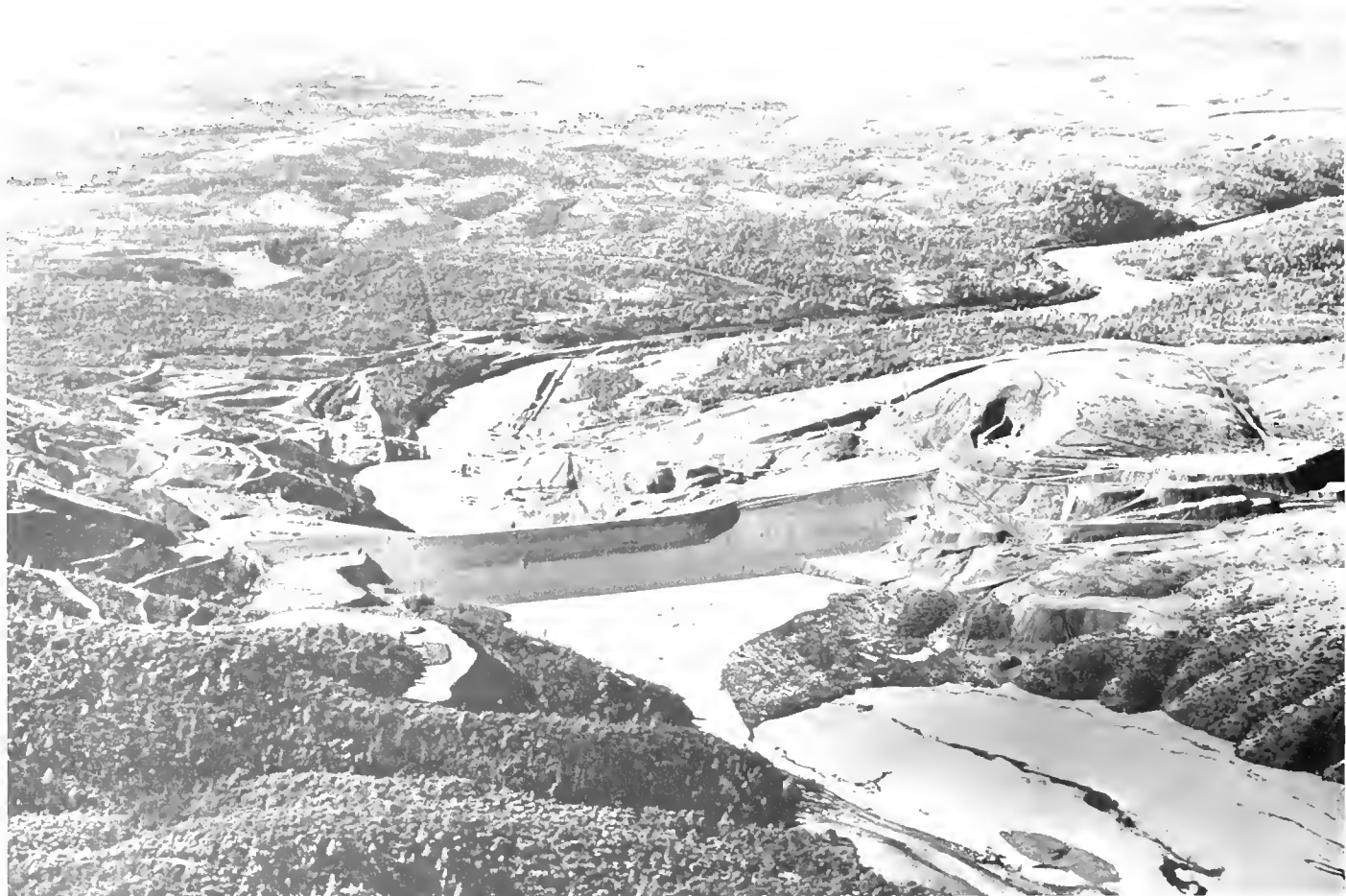
OROVILLE DAM, DECEMBER 24, 1964 CALIFORNIA DEPARTMENT OF WATER RESOURCES DATA ON PAGE 6
