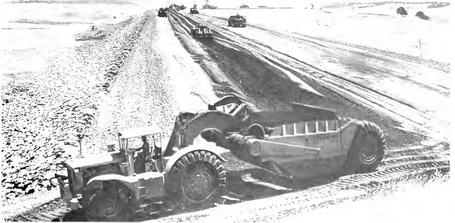
CAMANCHE DAM COURTESY BECHTEL CORPORATION DATA ON PAGE 64
