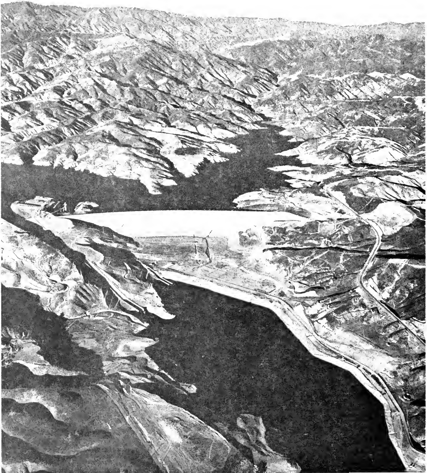
An aerial view of Castaic Dam and Reservoir, a terminal reservoir (capacity 350,000 acre-feet) of the State Water Project located in Los Angeles County about 40 miles north of the City of Los Angeles. The dam was completed in late 1973 and at the time of the photograph, December 11, 1973, the reservoir was filling. Castaic Lagoon (capacity 2,660 acre-feet) is in the foreground. (DWR photo No. 4411-72)
