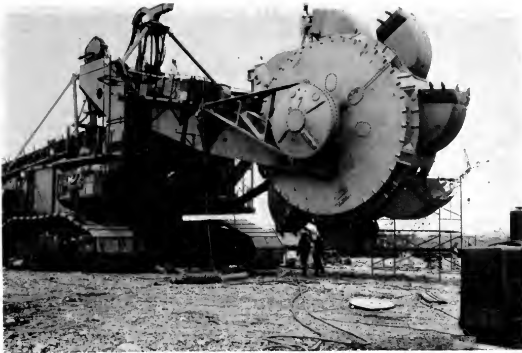
Dam construction in the 1960s and 1970s involved some very large mechanical equipment, as is evidenced by the bucket loader used at Oroville Dam and the sheepsfoot rollers and the carryall used at New Lake Arrowhead Dam.
