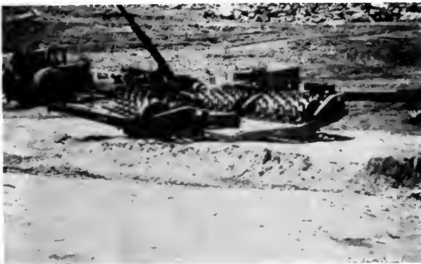
Dam construction in the 1960s and 1970s involved some very large mechanical equipment, as is evidenced by the bucket loader used at Oroville Dam and the sheepsfoot rollers and the carryall used at New Lake Arrowhead Dam.
