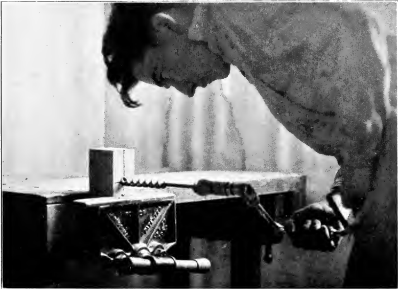
Fig. 156. Boring hole in head of mallet.
