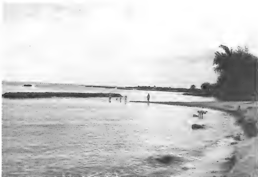
Figure 9. Breakwater at Haleiwa Beach, Hawaii (1966)
