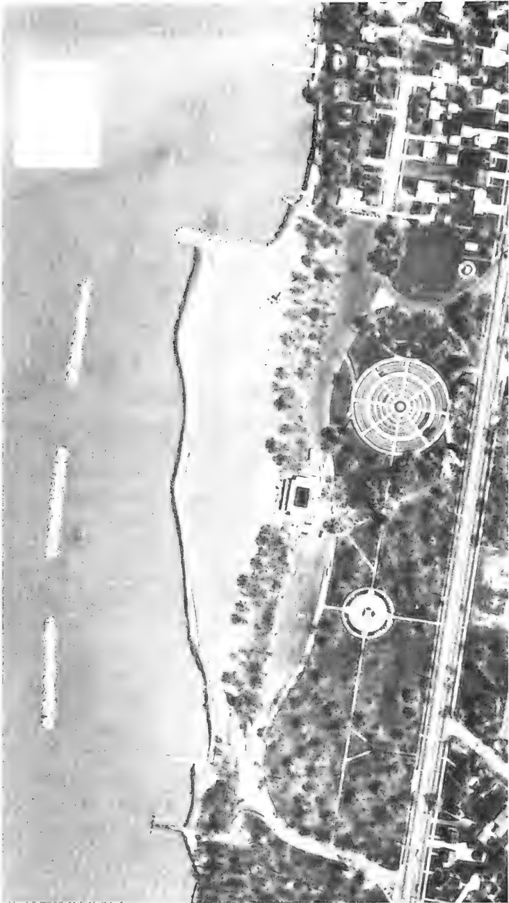
Figure C7. Aerial view of Lakeview Park showing the typical condition of the beachfill east of the west groin
