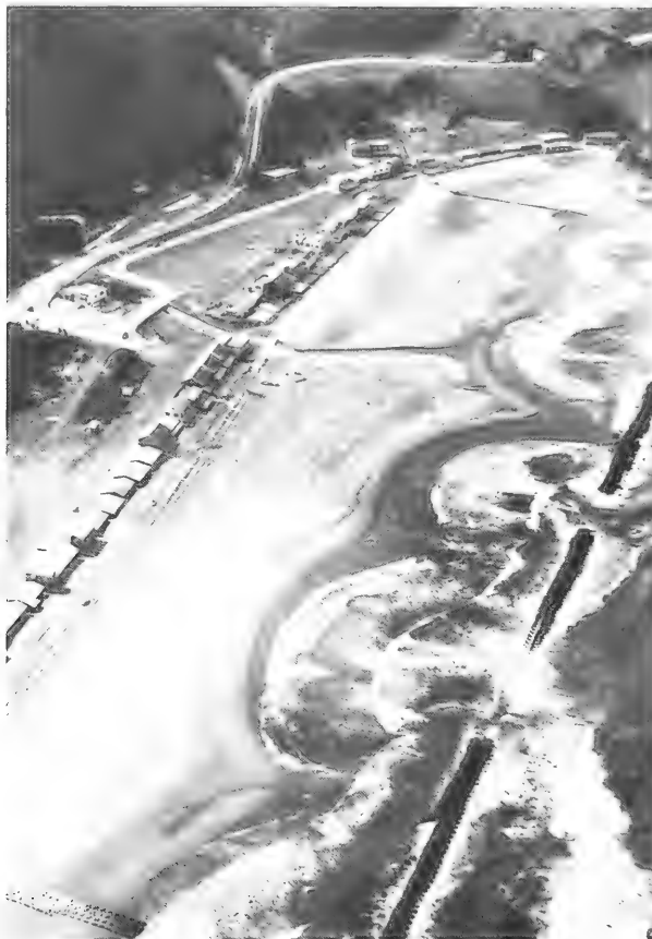
Figure 21. Permeable, overtopped, segmented breakwater located landward of breaker zone; Kakuda-Hama, Japan (1976)
