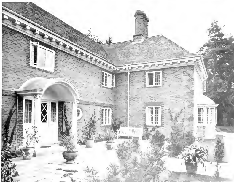
ARCHITECT: ST. J. NEWTON
