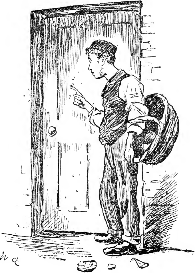
The grocer boy was actually picking off the paint on the side door, which had formed into blisters.
