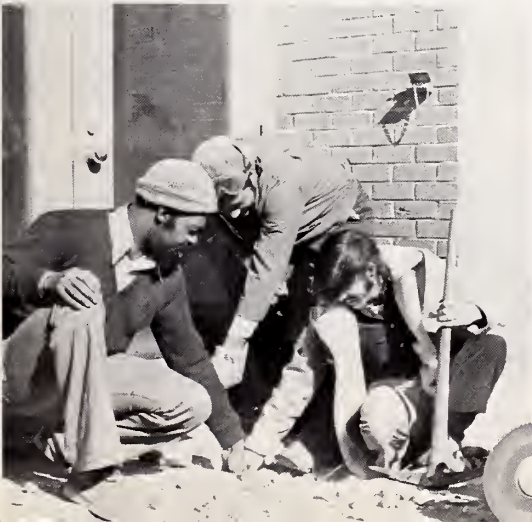
Masonry students remove old concrete while preparing to install a ramp for easier access to the building.
