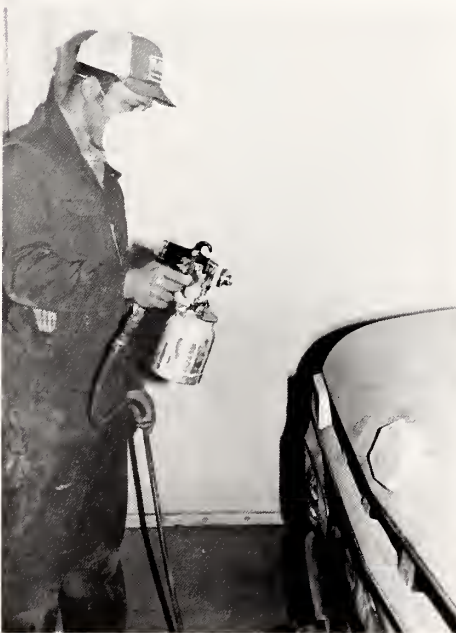
(above) Billy Ray Jacobs, Charles McLean and William Allen sand to prepare a car for painting. (left) Larry Ivey spray paints the primer surface.
