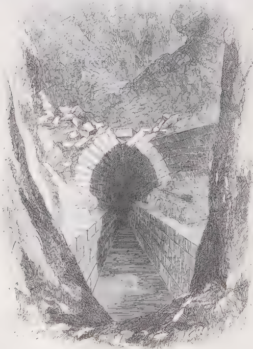
Vaulted Drain beneath South-east Palace (Nimroud)
