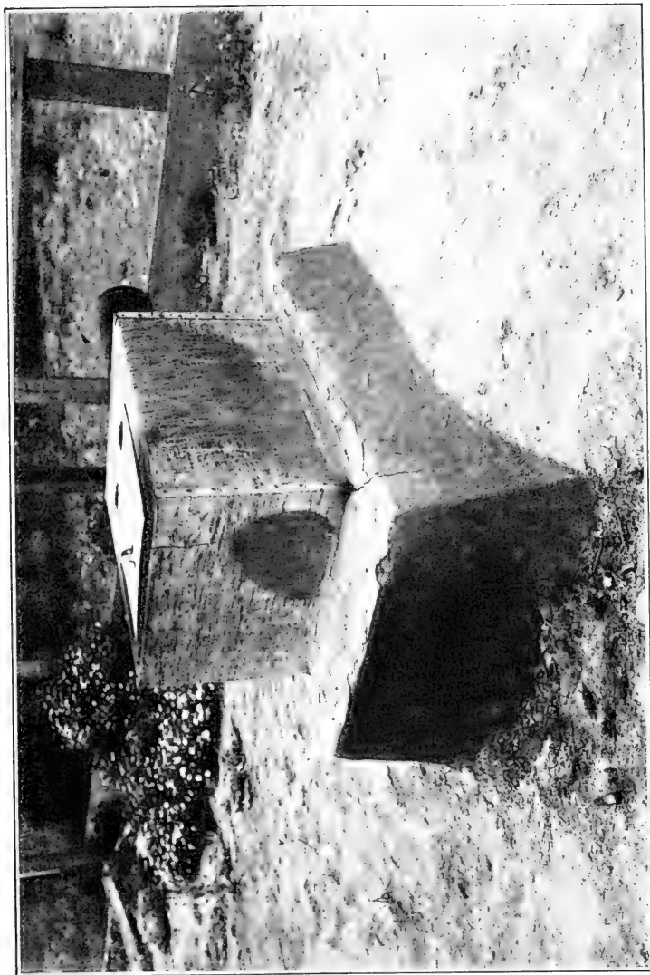
FIG. 5. — Photograph of crematory described in text. Note cement base, with opening in front into fire box; galvanized iron cremating box on top; cover of cremating box.
