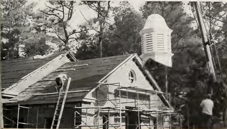
Construction workers lower cupola into correct position.
