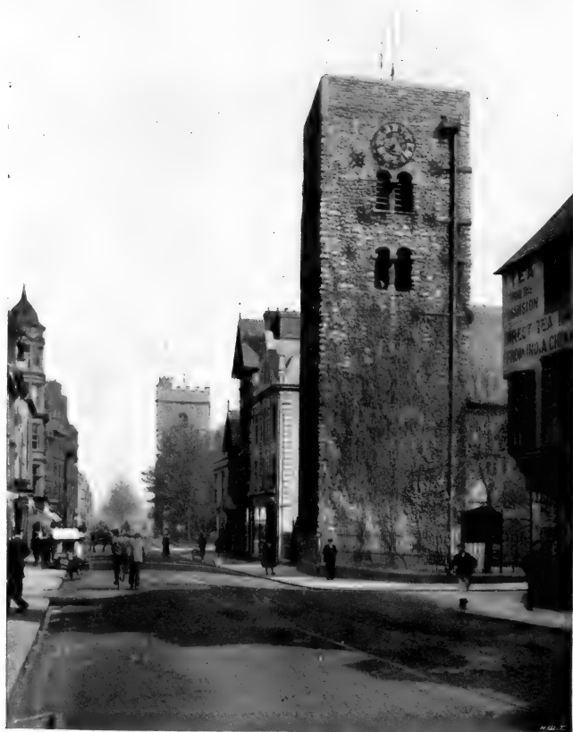
PRE-NORMAN TOWER (ST. MICHAEL'S, OXFORD)
