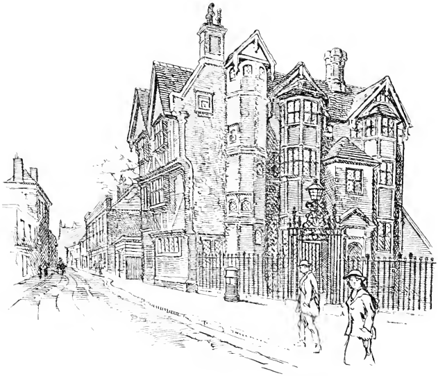
HIGH STREET, ROCHESTER: EASTGATE HOUSE.
