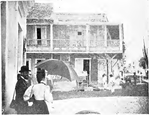
A Street Corner, Ponce.
