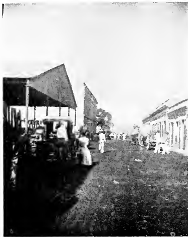
Street at the Bay, Ponce.
