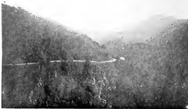
Improved Highway winding through the Mountains.
