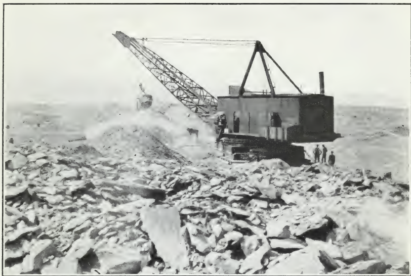
FIG. 1.—PRESSURE HAS CAUSED SHEARING ALONG BEDDING PLANES; WHEN EXCAVATED THE SHALE COMES OUT IN LARGE FLAKELIKE PIECES.
