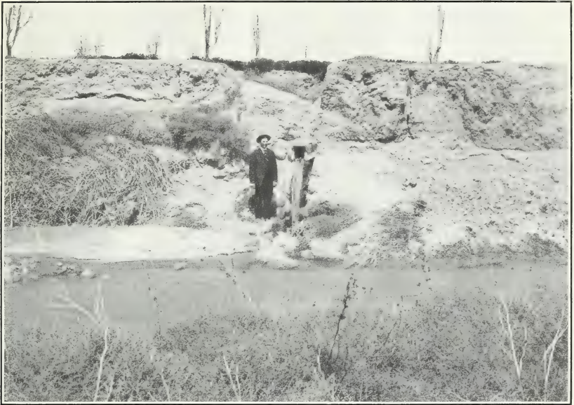
FIG. 1.—OUTLET OF DRAIN, SHOWING QUANTITY OF WATER DEVELOPED.
