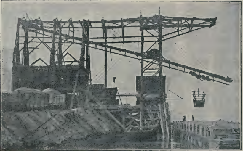
FIG. 79.—Machine for Unloading Sand from Barges.
