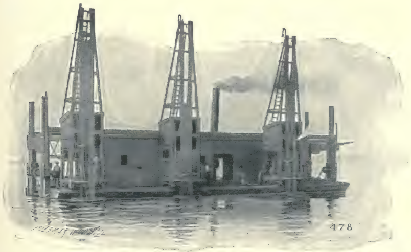
FIG. 7.—Ingersoll Drilling Scow.
