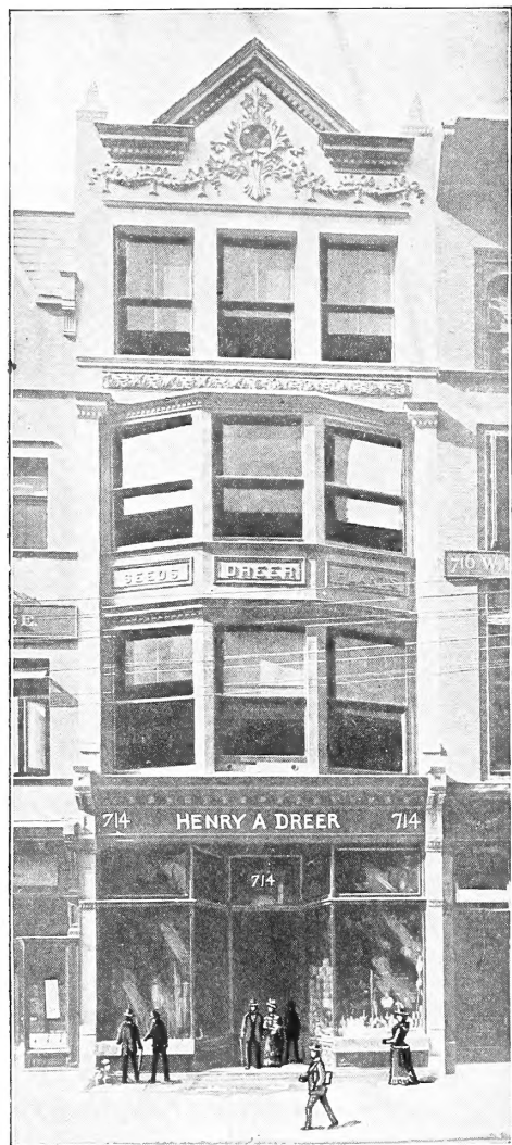
Present Store and Office, 714 Chestnut St.
