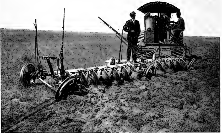
A GASOLINE-TRACTION PLOWING OUTFIT AT WORK ON A 3000-ACRE FARM IN MONTANA
