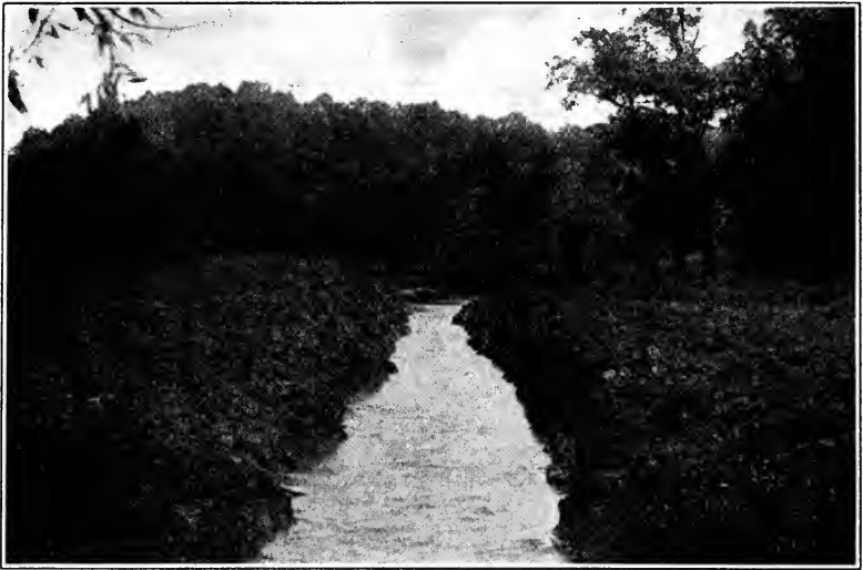
FIG. 23.—DITCH BLASTED AT WESTCHESTER, PA., TO CHANGE COURSE OF STREAM
