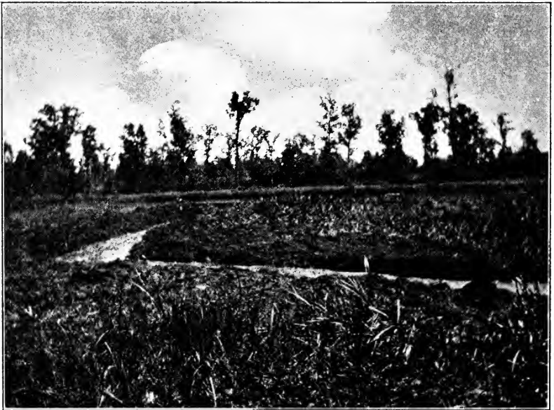
FIG. 22.—A DITCH BLASTED AROUND A CORNER IN ONE BLAST
