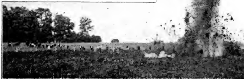
FIG 34 BLASTING THE POND SHOWN ON OPPOSITE PAGE
