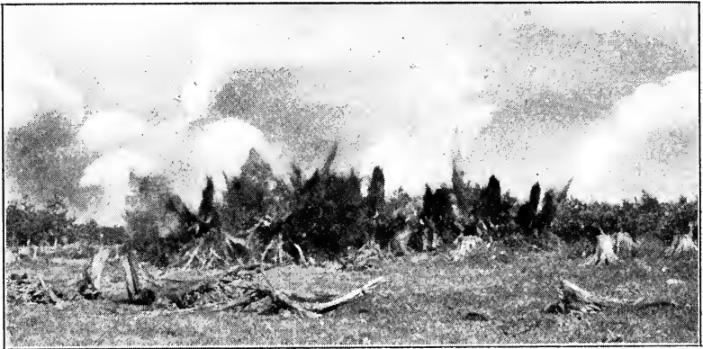
FIG. 15.—GROUP BLAST WITH BLASTING MACHINE, BARKSDALE, WIS.
