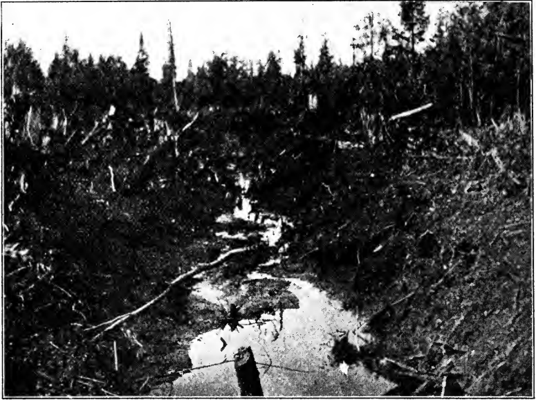
FIG. 21.—DYNAMITING DIGS DITCHES THROUGH LAND THAT CANNOT BE ECONOMICALLY HANDLED OTHERWISE
