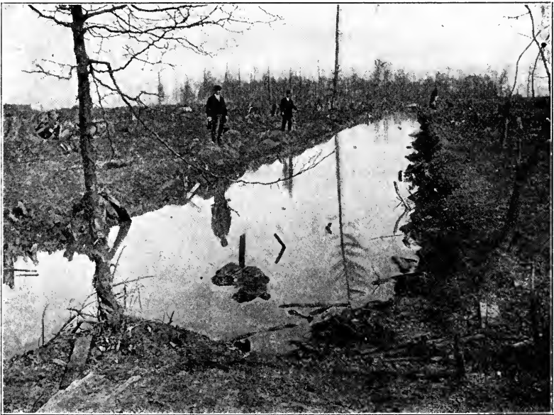
FIG. 29.—SAME DITCH AS IN UPPER VIEW, FILLED
