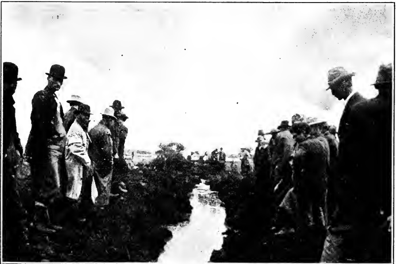
FIG. 24.—DITCH BLASTED IN HEAVY SOIL AT ALBANY, ORE.
