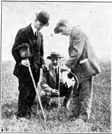
FIG. 111 LOWERING PRIMED CARTRIDGE INTO HOLE
