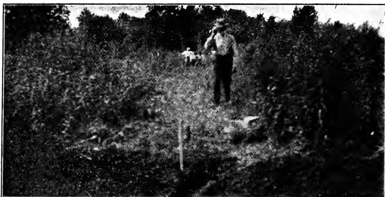
FIG. 25.—BEFORE THE BLAST, BURKETT FARM, NEWBURGH, N. Y.
