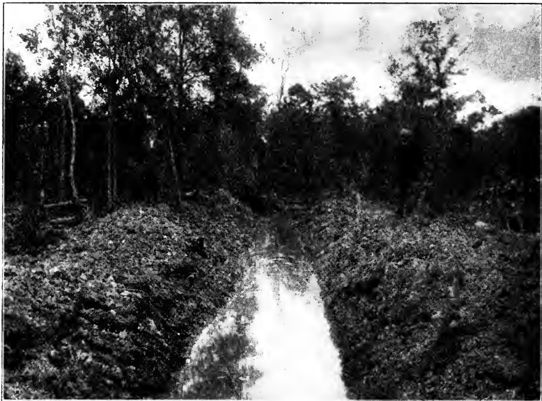
FIG. 19.—GOVERNMENT EXPERIMENT IN BLASTING DITCHES, CHARLESTON, S. C.
