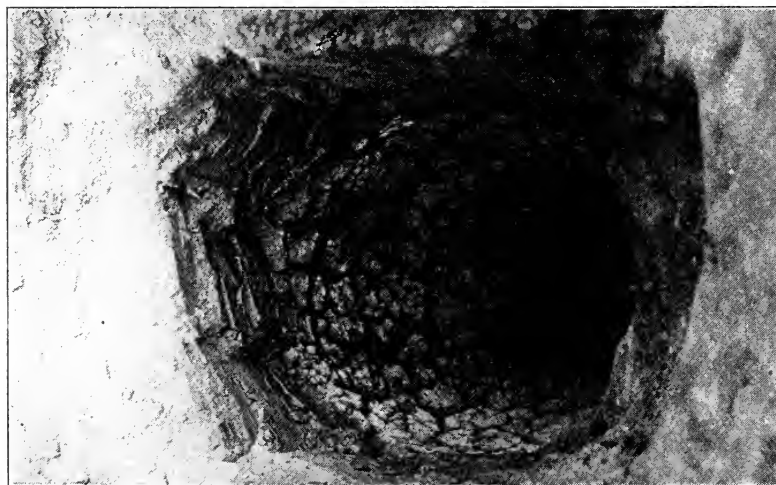
FIG. 41.—TOP OF HOLE BLASTED FOR PLANTING FRUIT TREE. (NOTE RADIAL FISSURES)
