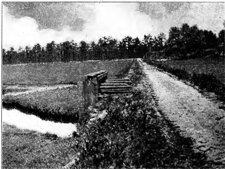
FIG. 30.—DITCH BLASTED WITH DYNAMITE. RIDER CRANBERRY BOGS, HAMMONTON, N. J.
