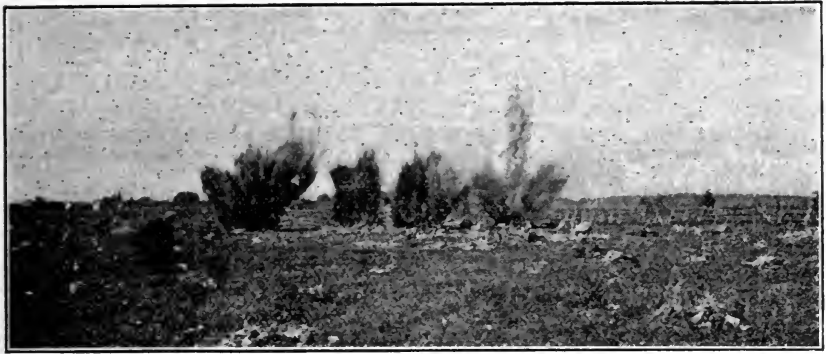
FIG. 117.—BLASTING STUMPS ELECTRICALLY
