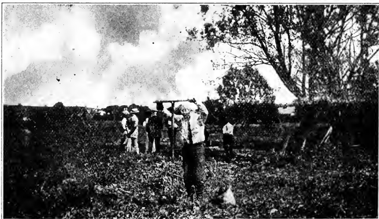
FIG. 118A.—MAKING HOLES WITH PUNCH BAR
