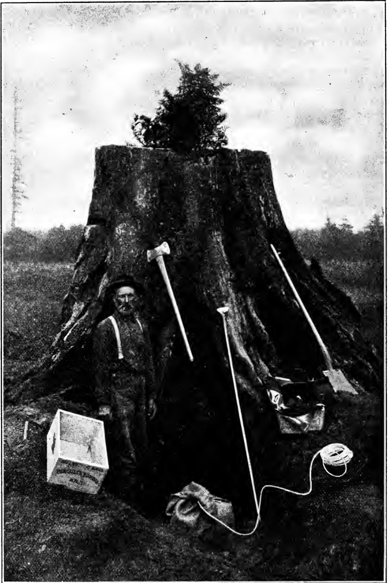
FIG. 127.—ILLUSTRATING METHOD OF PLACING CHARGE UNDER A CALIFORNIA BIG-TREE
