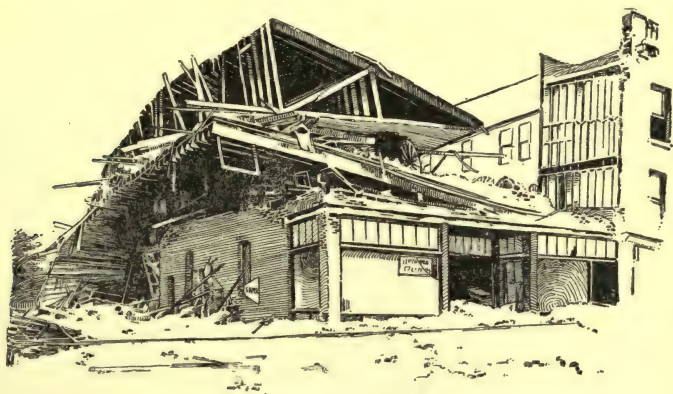
FIG. 86.—Building wrecked at San Mateo, California, during the late earthquake. The heavy roof and upper floor, acting as a unit, have battered down the upper walls (after J. C. Branner).
