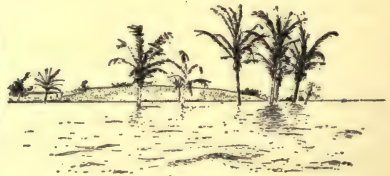
FIG. 75.—Settlement of a section of the shore at Port Royal, Jamaica, during the earthquake of January 14, 1907, adjacent to a similar but larger settlement of the near shore during the earthquake of 1692 (after a photograph by Brown).
