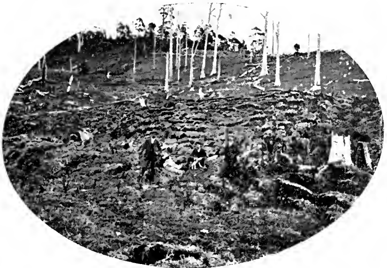
THE LANDSLIP, BREAM CREEK.
