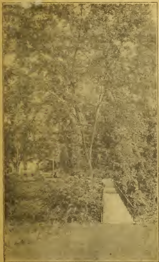
Footbridge over Chico Creek, Bidwell Grounds
