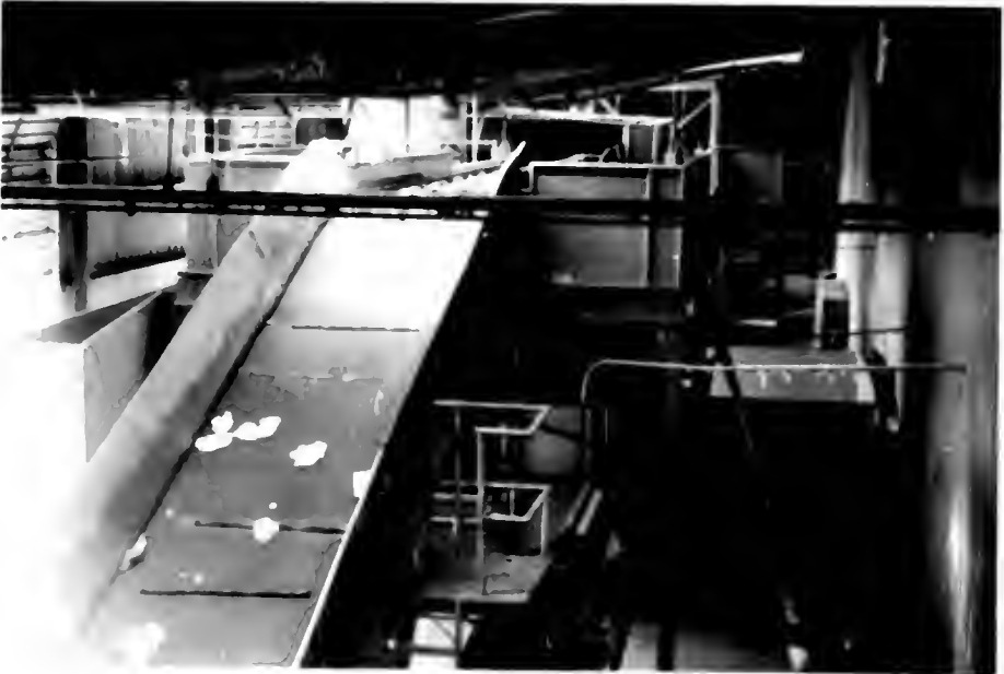
Fig. 4. Sorting conveyor carries refuse to sorting platform.
