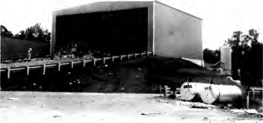
Fig. 3. Receiving building filled with refuse.
