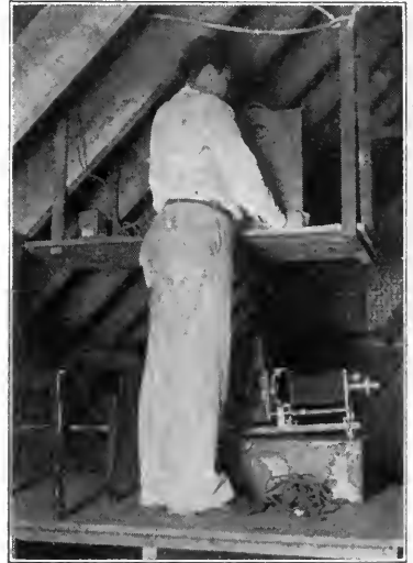
Runway behind stage. Platform built over old ventilating shaft. Projection through old register opening in rear wall of stage.
