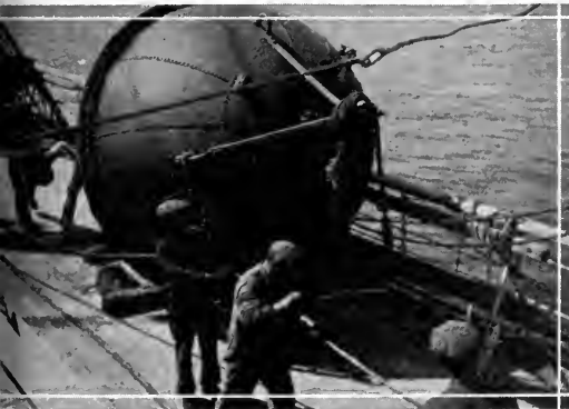
Splicing the cable on board the "Colonia"
