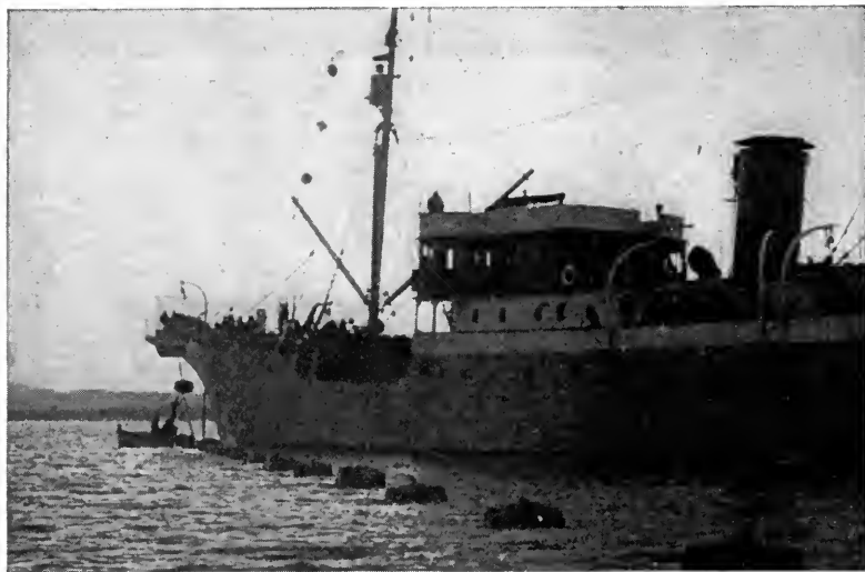
Air-tight barrels float the wriggling serpent-like cable in to the beach.
