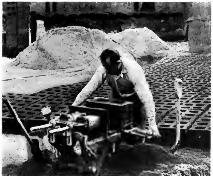
Making sandstone blocks—from the Eastman classroom film, "Sand to Clay."
