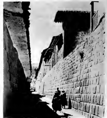
An Inca Wall in Cuzco
