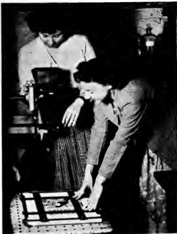
Copying, using plate-back camera with double extension bellows.
