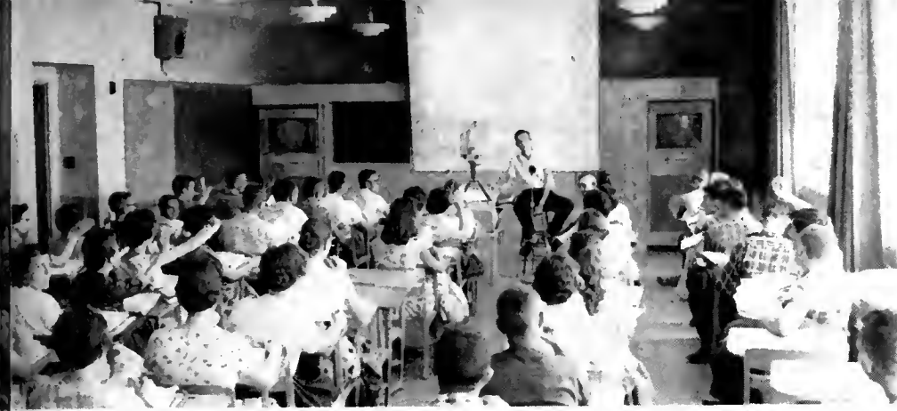
A typical large-class session in Snyder, Texas. Closed circuit TV, rear-projection equipment, a magnetic board and a large tilted viewing screen have been arranged in a panel located three feet from the front wall.
