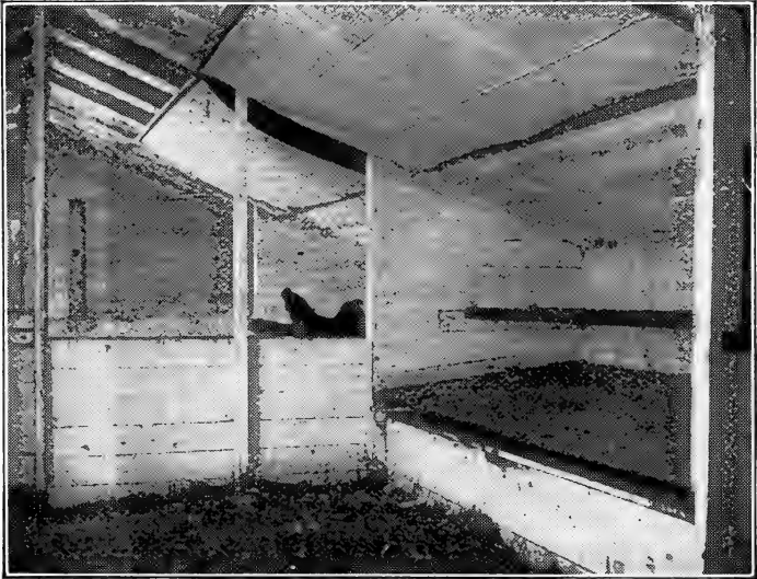
Interior of a House for Winter Layers, Showing the Roost and Roost Platform with Curtain to let Down in Front.
