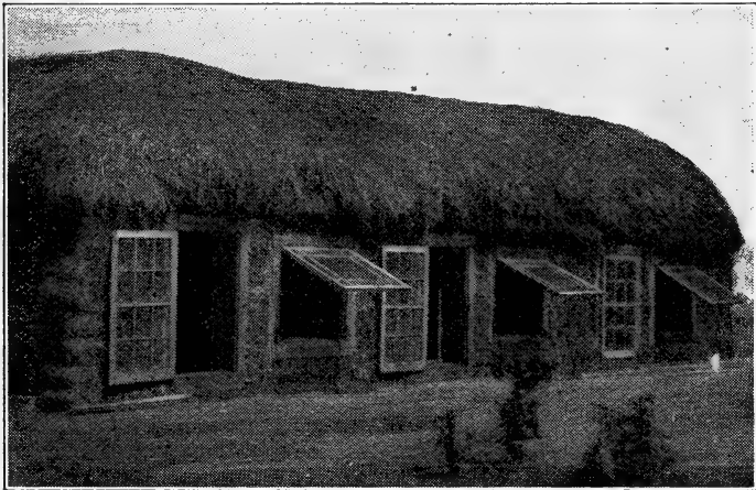
Winter Quarters for a Farm Flock, Built Almost Entirely of Straw, Baled or Loose.
