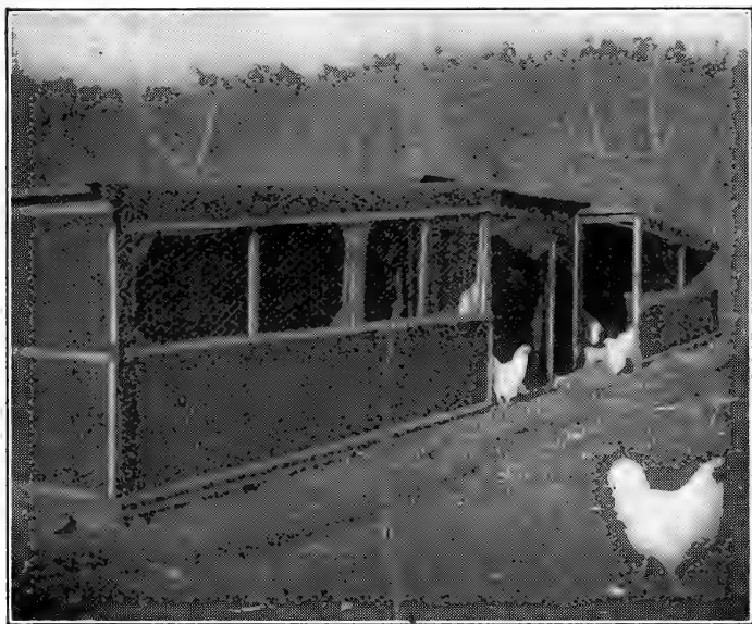
A Poultry House Consisting Only of Frame Covered with Tar Paper, with a Central and Warmer Roosting Pen.
