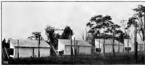
Row of Colony Houses at West Virginia Experiment Station; Rear View.
