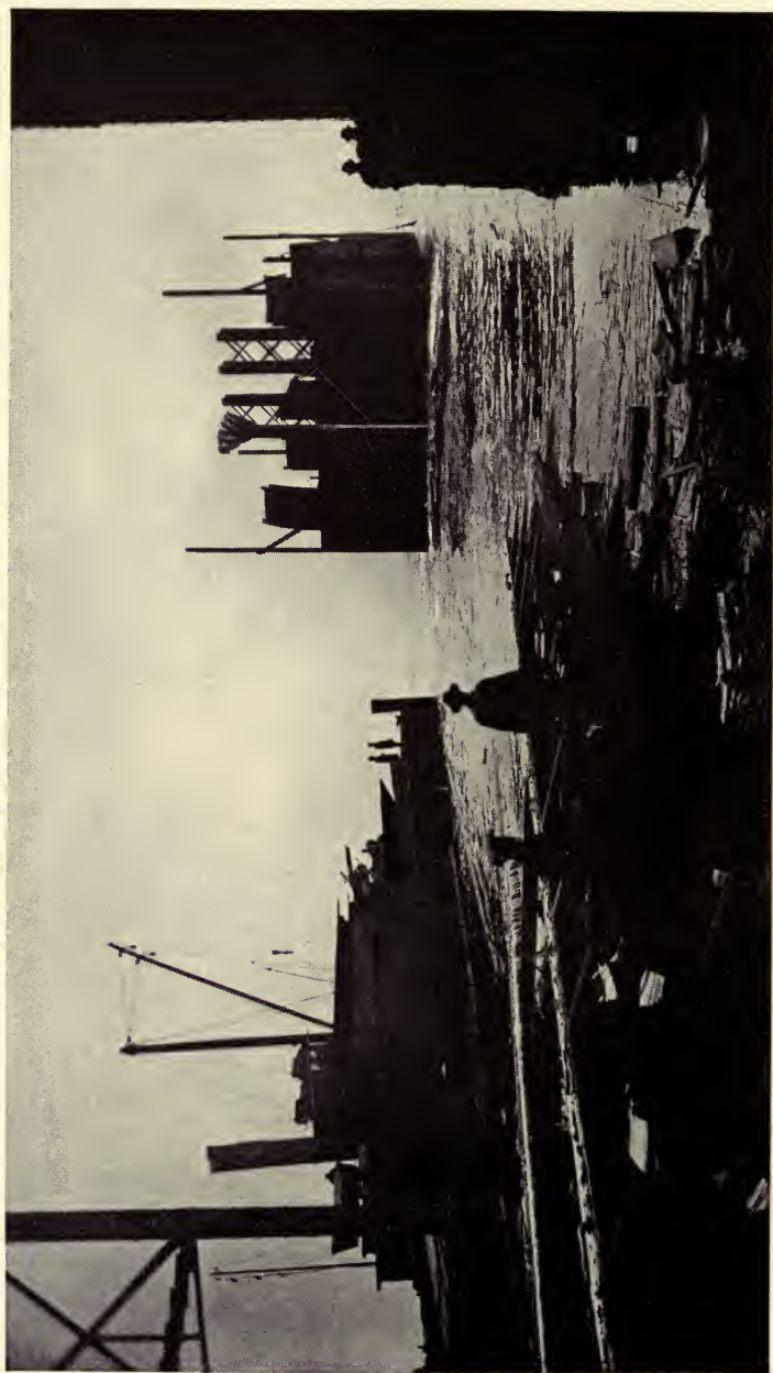
NEW JERSEY RIVER SHAFT CAISSON, JUST AFTER LEAVING THE WAYS Caisson launched at Mariner's Harbor, Long Island, floated into position and sunk
