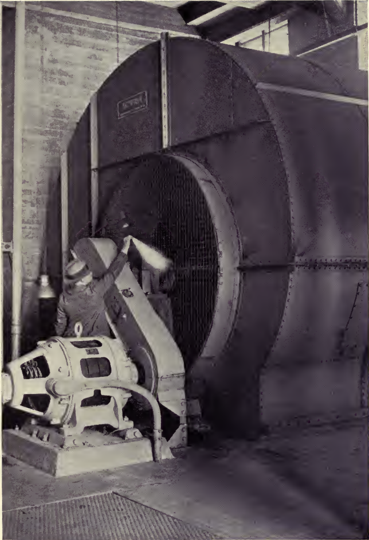
ONE OF THE 84 STURTEVANT SILENTVANE FANS Which are the lungs of the Holland Tunnel
