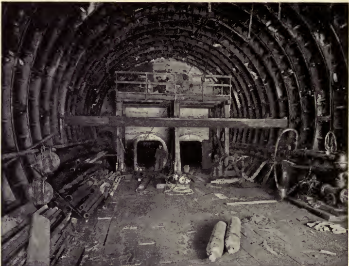
CONCRETE BULKHEAD AND LOCKS South Tunnel, Canal Street, New York City
