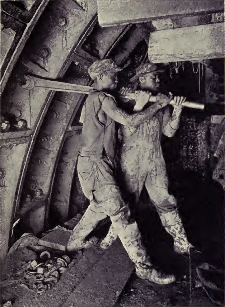
TIGHTENING BOLTS IN TUNNEL LINING, NORTH TUNNEL By means of ratchet wrench. Each bolt weighs ten pounds
