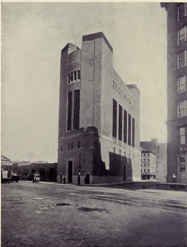
LAND VENTILATION BUILDING West side of Washington St., Canal to Spring Sts., New York City
