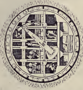
REAR OF SHIELD ERECTION OF IRON & MUCKING IN PROGRESS
