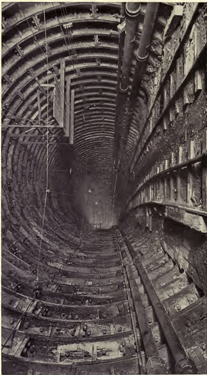
CURVE IN SOUTH TUNNEL UNDER WEST STREET, NEW YORK CITY (RADIUS 1000 FEET) Showing completed rings of cast-iron lining
