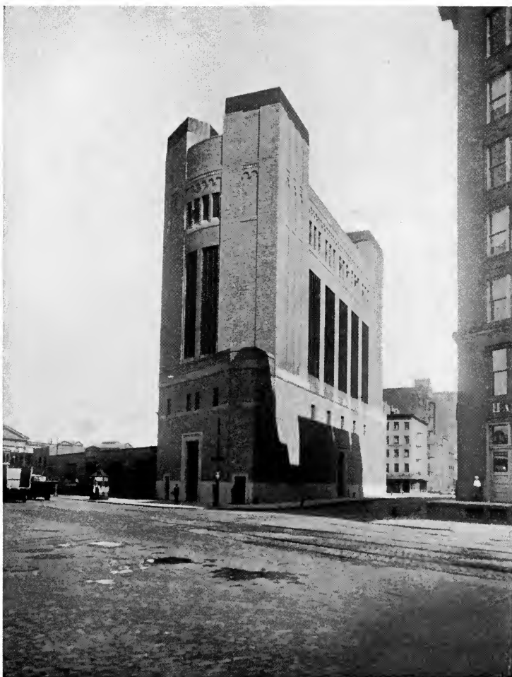
LAND VENTILATION BUILDING West side of Washington St., Canal to Spring Sts., New York City
