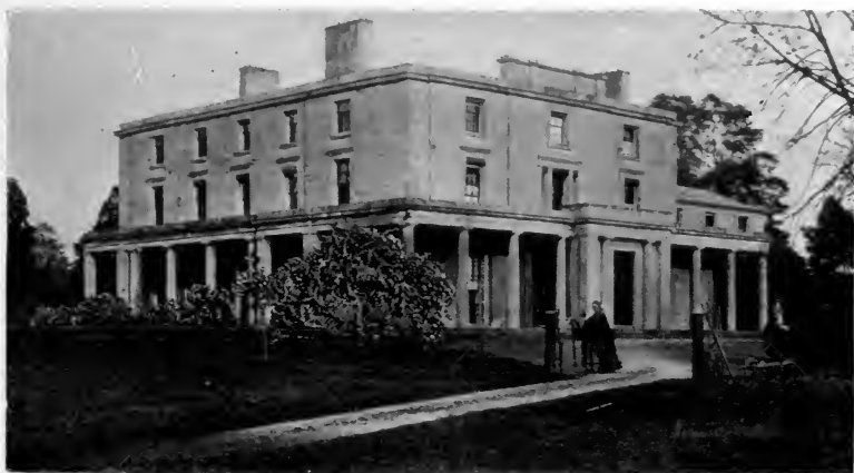
MANSION HOUSE, SEDBURY PARK; MISS GEORGIANA ORMEROD ON THE LEFT, MISS ELEANOR ORMEROD ON THE RIGHT.
