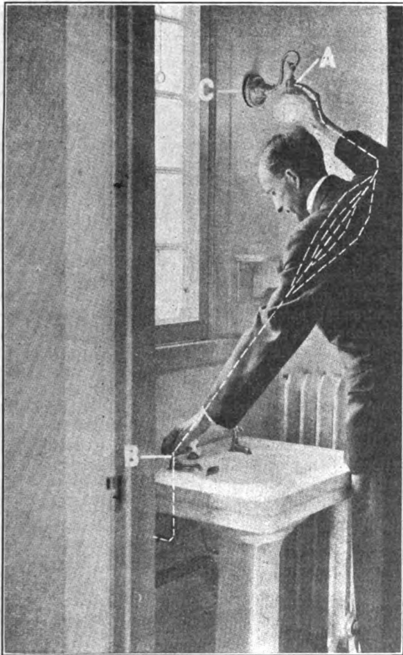
Fig. 2.—Illustrating danger from shock when in contact with an electrical fixture having an exposed metal frame which is not grounded.
