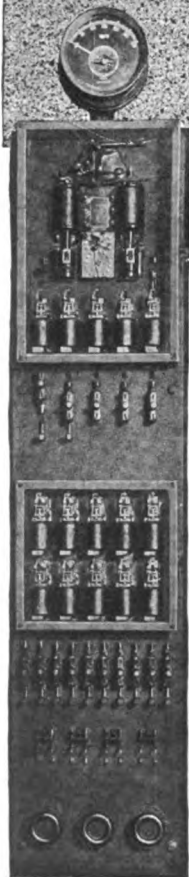
Fig. 1—Type AN-12 Generator Voltage Regulator for Controlling Three Exciters, Each Connected Directly to a Generator with Generators in Parallel Eastern Michigan Power Co.'s 18,750 K. V. A. Junction Development.
