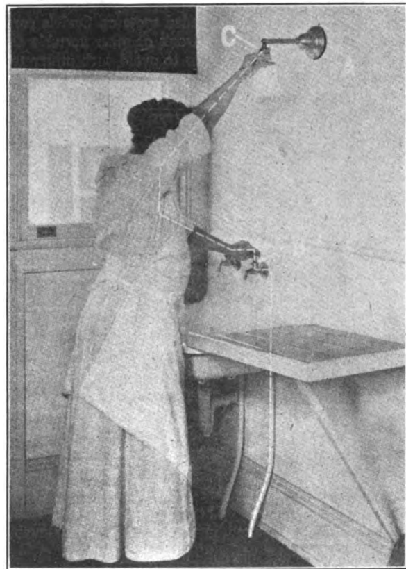
Fig. 8.—Illustration of the possible danger from shock by the passage of electricity from the metallic undergrounded fixture C . (see insulating ring at base of fixture A .) through the body to the grounded water faucet at B .
