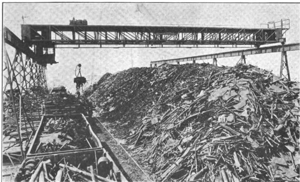
Fig. 7-A. Outdoor traveling crane
