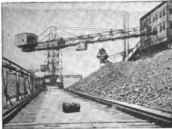
Coal handling crane installed at the La Belle Iron Works plant at Steubenville, Ohio.
