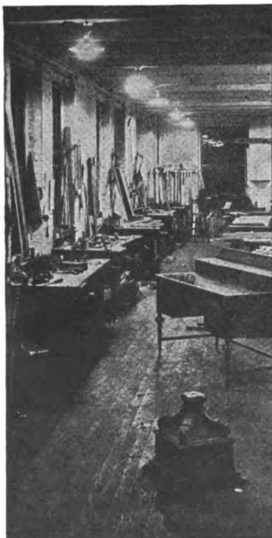
Fig. 6. Lighting installation over benches (problem 3.)
