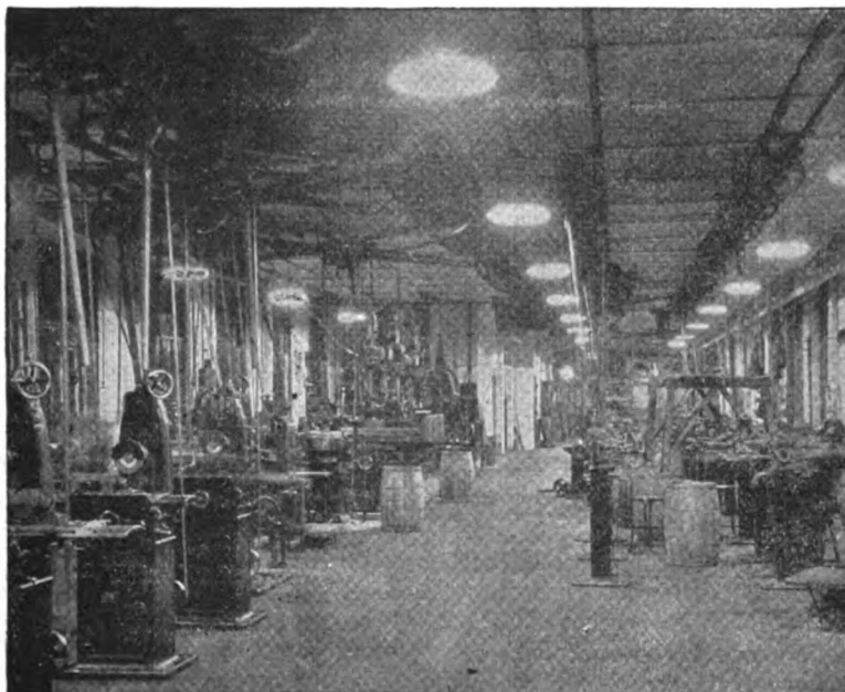
Fig. 10. Installation of metal-working plant (problem 4)
