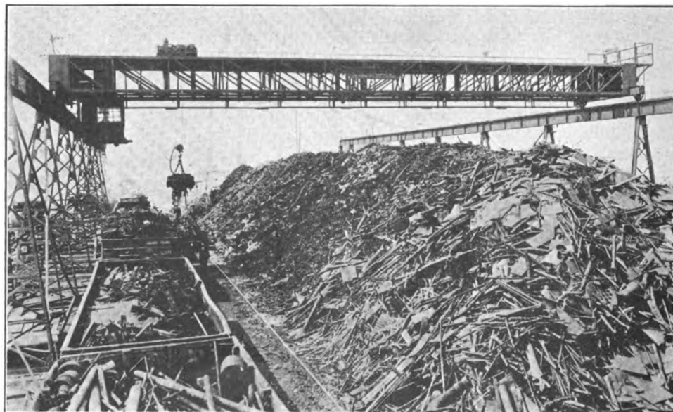
Fig. 7-A. Outdoor traveling crane
