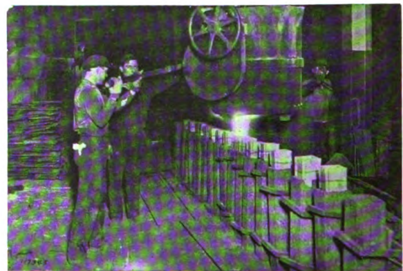
FILLING MOULDS FROM ELECTRIC FURNACE
