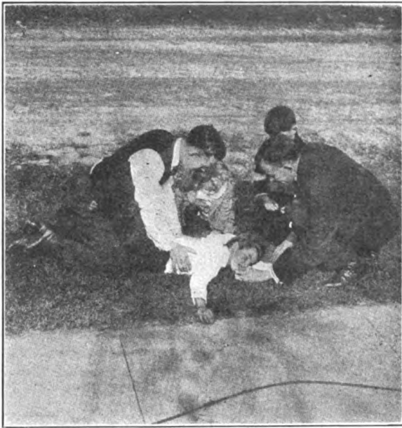
Fig. 1.—The prone-pressure method of resuscitating a person who has received an electric shock.
