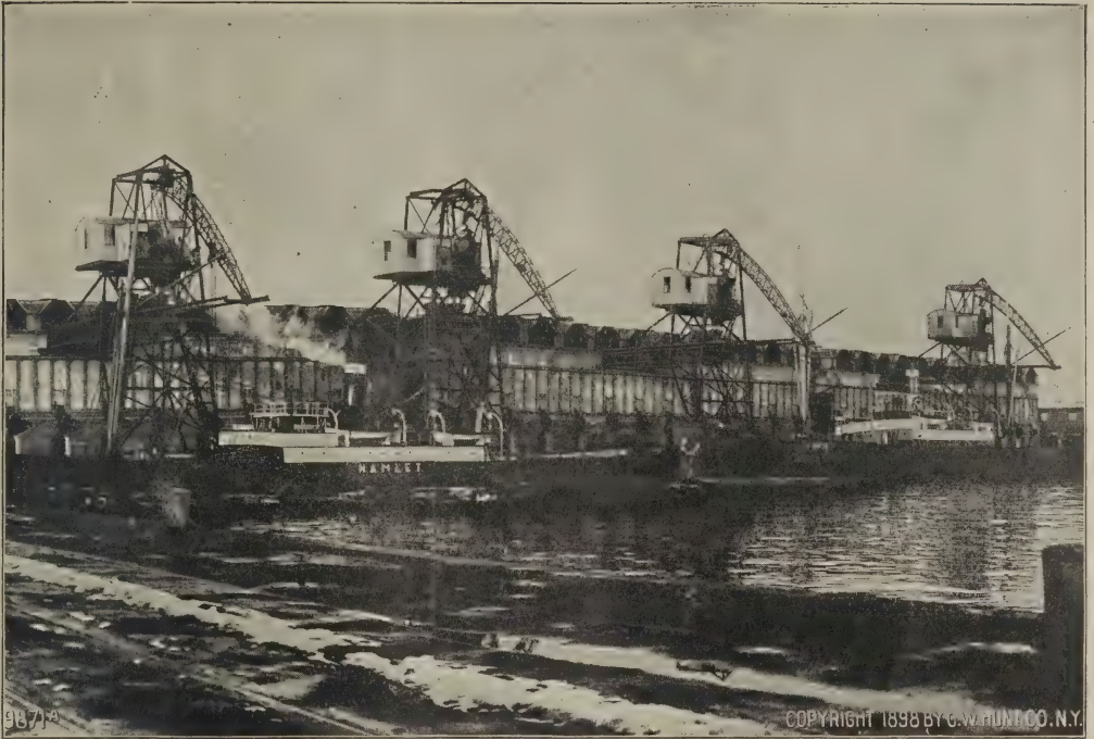
American Elevators at Work at the Wharves of the Danish Coal Company.
