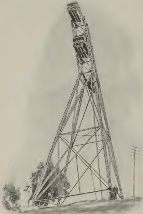
Leaning Tower of the Carquinez Span.
