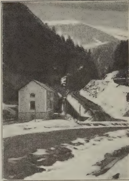
Railroad Power House in the Ravine of Chatclard.
