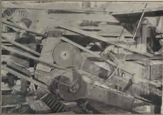
Apparatus for Transferring the Shoes from their Temporary to Permanent Positions.
