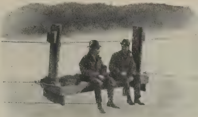
Overhead Cableway Across Yuba River.
