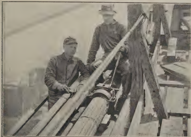
Squeezing and Binding the Core of the Cable in Midair
