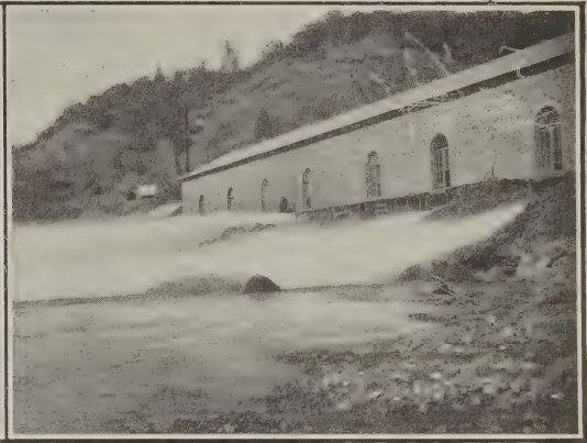
Outflow at Light Load. The Stream Sometimes Shoots Across the Cañon; It Does Not Strike the Buckets and Is Uncontrolled.
