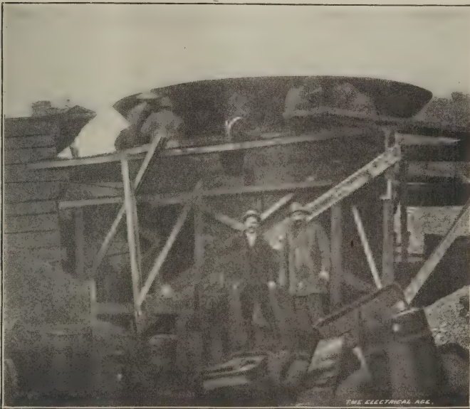
Constructing the Mouth of the Compressor.
