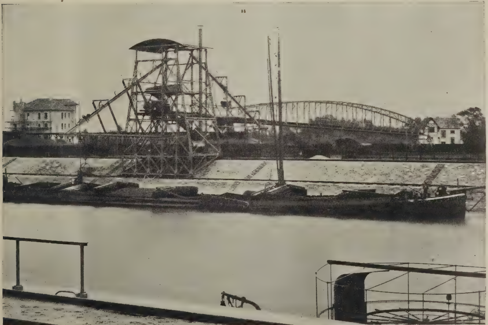
Hunt Elevator and Automatic Railway erected for the Rheinisch-Westfaelisches Kohlen-Syndicat, at Ludwigshafen, Germany.
