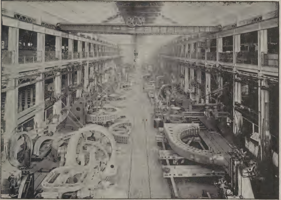
Main Aisle, Westinghouse Electric and Manufacturing Company's Works, East Pittsburgh, Pa.
