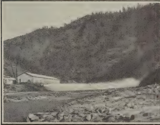
Outflow at Light Load. The Stream Sometimes Shoots Across the Cañon; It Does Not Strike the Buckets and Is Uncontrolled.
