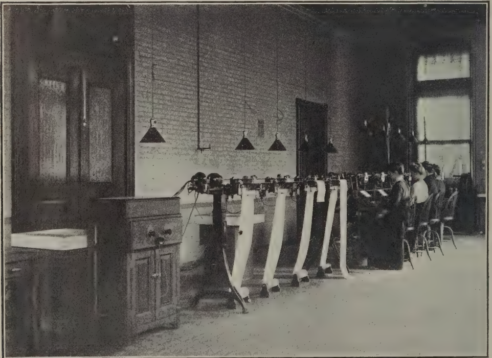
Four Messages Being Sent at Once from One End of a Single Wire and Home Recorders Making Duplicate Copies.
