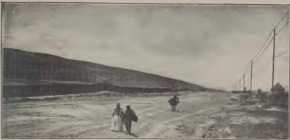
The Bogota High Tension Transmission Line Between Power Plant and City. The Line is Sixteen Miles Long.
