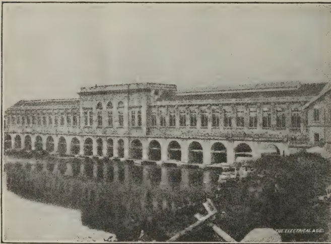
Exterior View of the Power House of the Cusset Works, Jonage.
