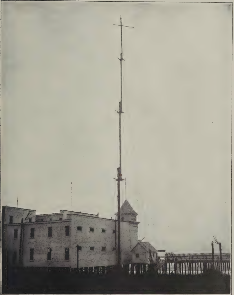
Coney Island, New York City, Mast and Station, de Forest Wireless Telegraph Company. Height of Mast, 210 feet. The Antennae Descend from the Yard-Arm to the Small House which Contains the Station.
