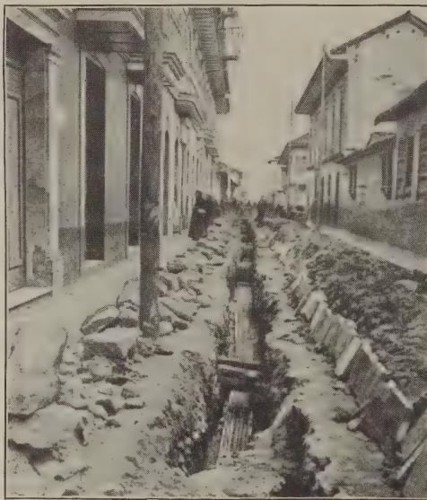
High Tension Power Transmission Cables in Conduits at Bogota.
