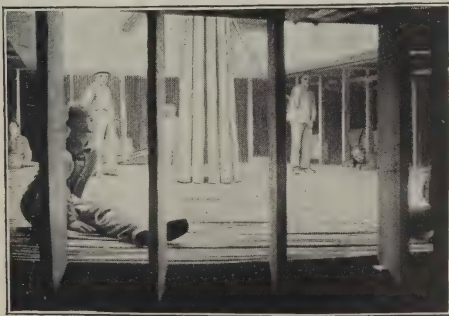
Interior View of Cable-Tank, S.S. Lakme .
