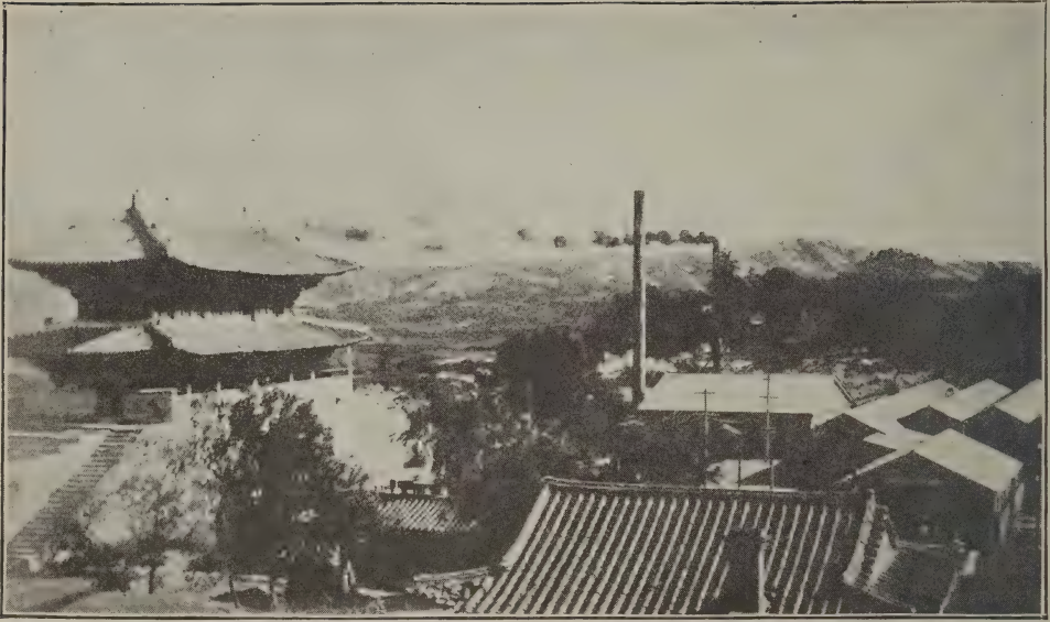
Power House of the Seoul Electric Company, Seoul, Korea.—The Largest Electric Plant in Asia.
