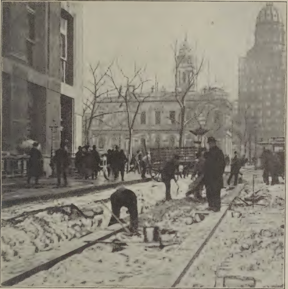
Laying the New Steel Roadway in Murray Street, New York. Constructed by General Roy Stone, under the Auspices of the Automobile Club of America.
