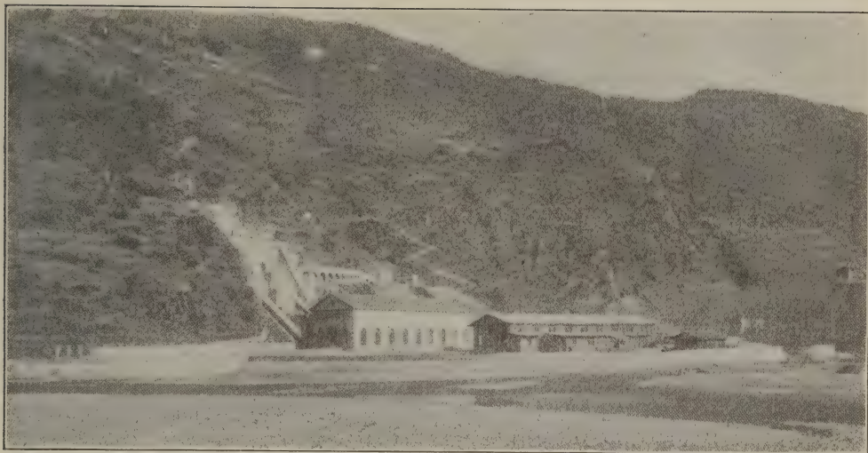
Power House at Morbegno, Italy, of the Valtellina Railway.
