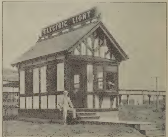
The "Electric Cottage."
