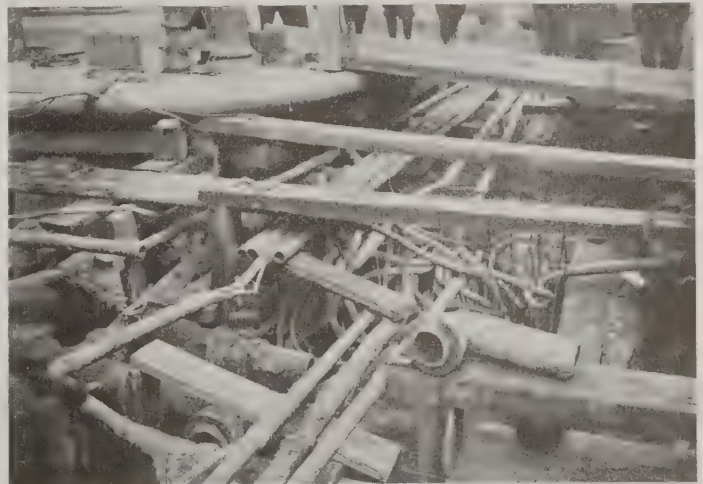
N. W. Corner Broadway and Broome Streets. Manhole Under Construction.
