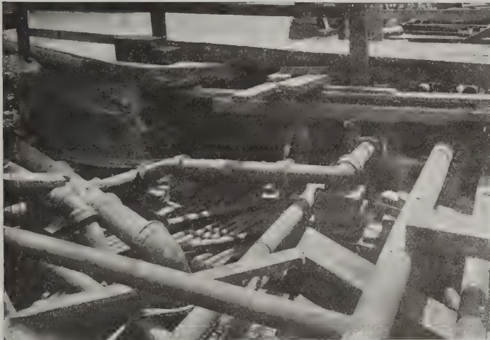
Broadway and 27th Street. Iron-Pipe Telephone Ducts Below Other Pipes
