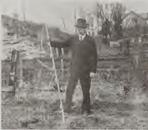
The Charge Ready to be Placed
