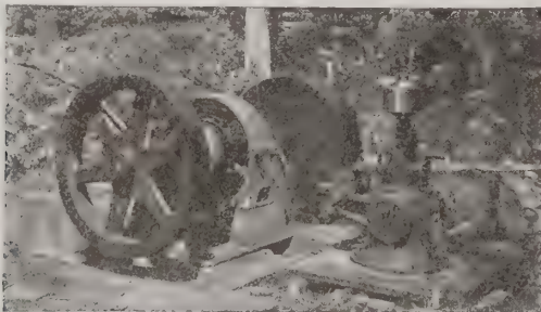
An impulse-wheel outfit in course of installation. This wheel is made by the Pelton Water Wheel Co., New York and San Francisco.
