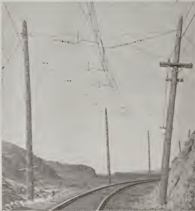
Typical Overhead Construction on a Curve
