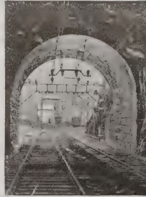
The Tunnel Portal
