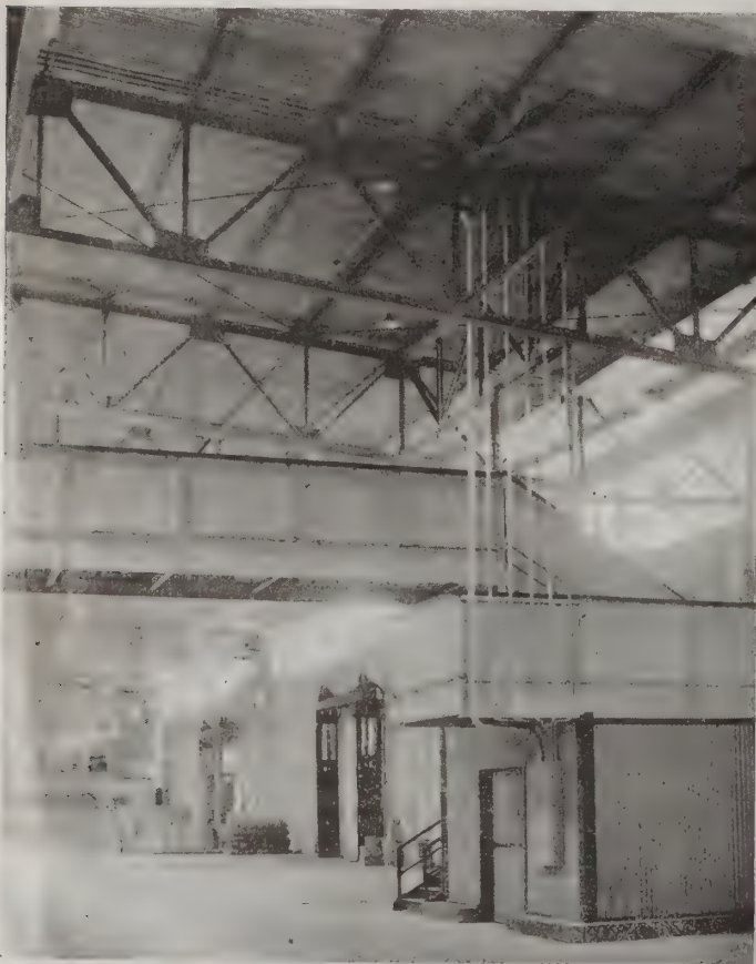
Fig. 1. Interior of Pier
