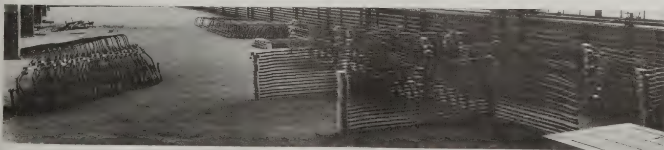
Fig. 7. Conduits bent and fitted ready to be put in place.
