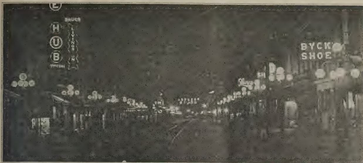
FIG. 8. BROUGHTON STREET AT SAVANNAH.
