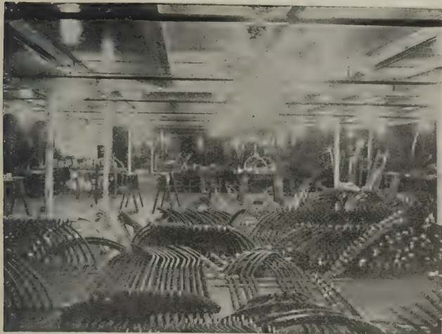
FIG. 3. FACTORY WITH LOW CEILING WHERE 60-WATT TUNGSTEN LAMPS HAVE BEEN A SUCCESS.
