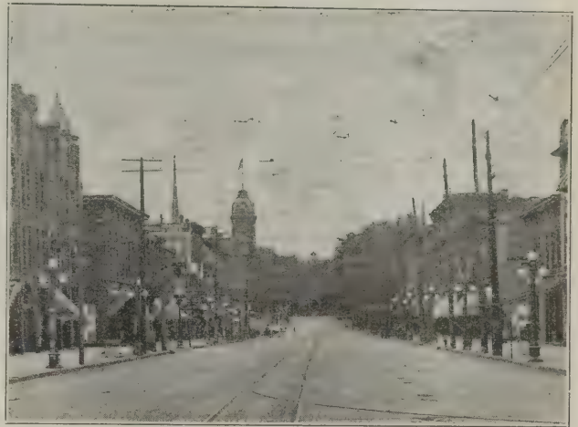
FIG. 2. THREE-LIGHT DECORATIVE SYSTEM, WARREN, OHIO.
