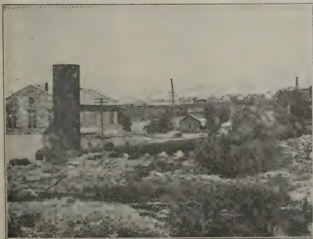
FIG. 1. VIEW OF POWER HOUSE, SHOWING PIPE LINE AND SURGE TANK.
