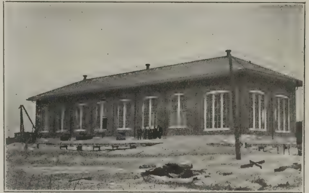
FIG. 2. PUMPING STATION BUILDING.
