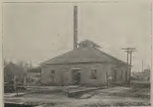
FIG. 2. MONROE ELECTRIC PLANT.
