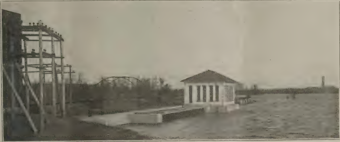
FIG. 9. HYDRO-ELECTRIC PLANT AND DAM AT LOWELL. TRANSFORMER HOUSE AT LEFT, RIVERTON STATION IN DISTANCE AT RIGHT.
