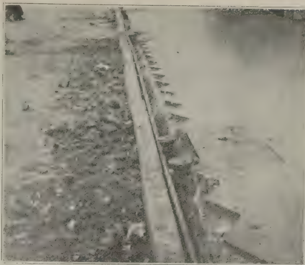
FIG. 3. LAYING OF CONDUIT IN CURB.
