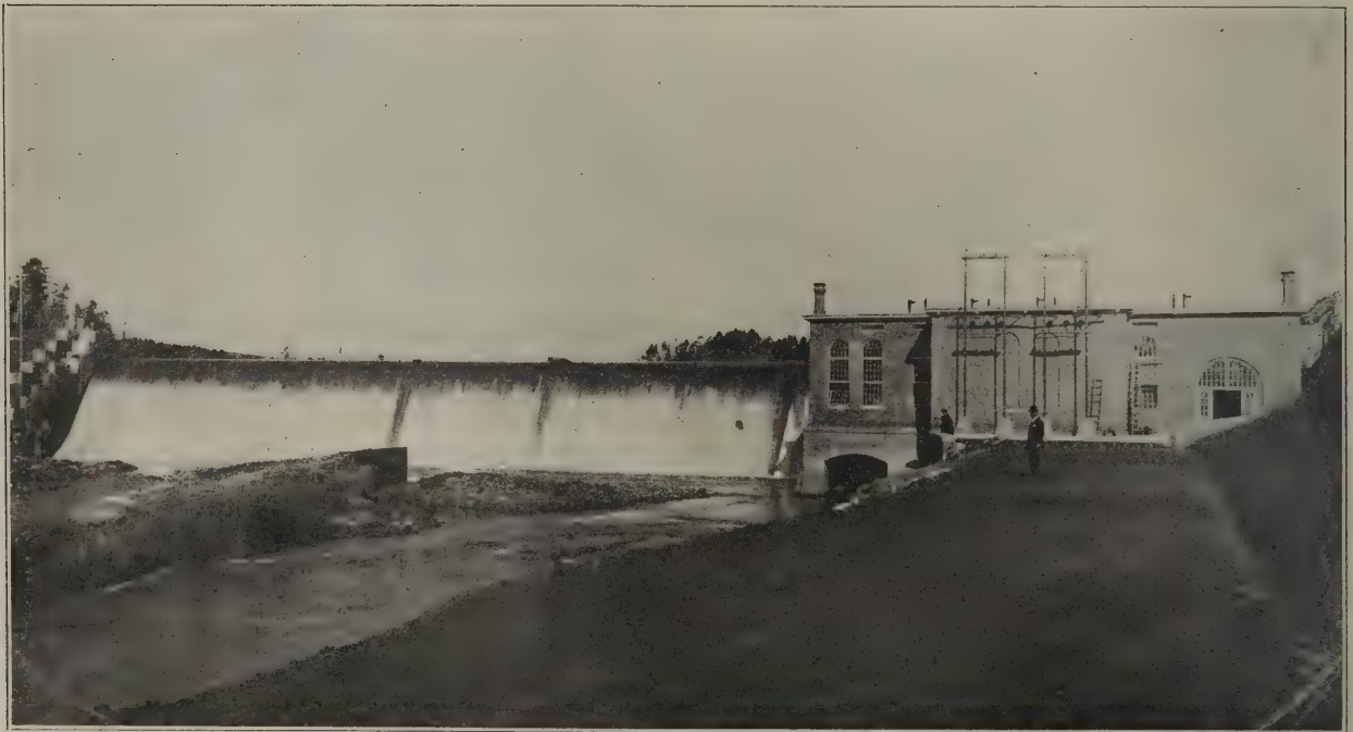
FIG. 1. HYDRO-ELECTRIC DEVELOPMENT ON SALUDA RIVER.
