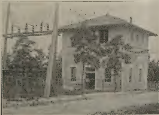
FIG. 1. SUBSTATION OF SOUTHERN POWER COMPANY.
