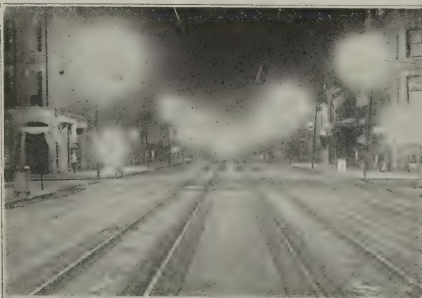
FIG. 10. REGENERATIVE FLAME ARC SYSTEM AT PUEBLO, COL.
