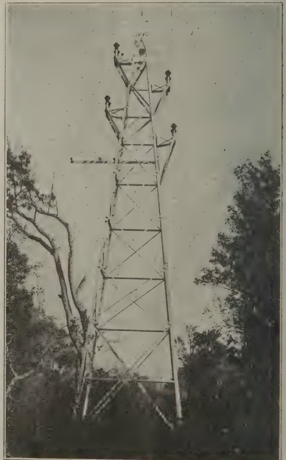
FIG. 8. TOWER FOR 33,000 VOLT LINES AT CROSSING POINT OF SPRING RIVER.
