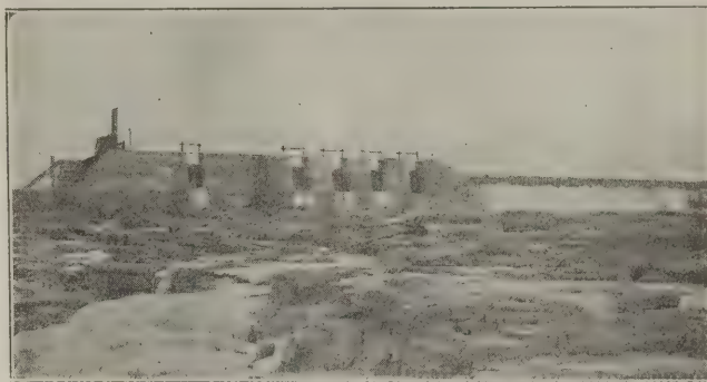
FIG. 2. VIEW OF DAM.
