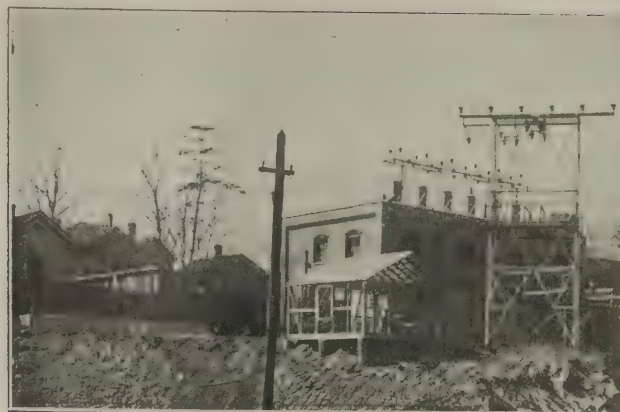
FIG. 9. EXTERIOR OF MACON SUBSTATION SHOWING INCOMING 66,000 VOLT LINES.
