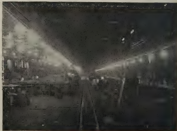
FIG. 2. FACTORY WHERE 100-WATT TUNGSTEN LAMPS GIVE A UNIFORM ILLUMINATION.
