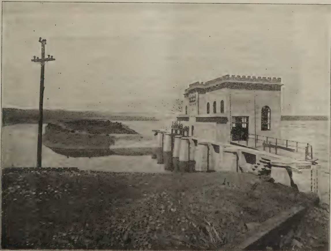
FIG. 4. EXTERIOR OF POWER HOUSE SHOWING NATURE OF DEVELOPMENT.
