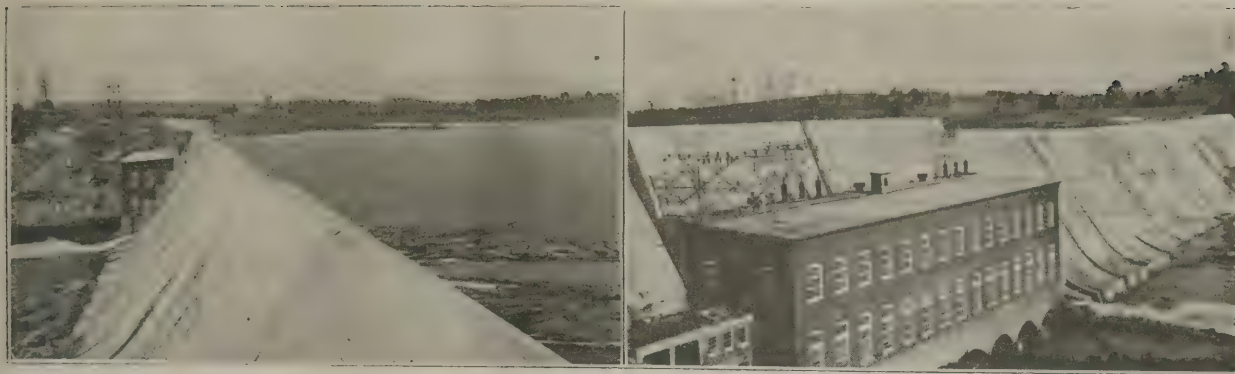
FIG. 2. GENERAL VIEW OF POWERHOUSE, OUT GOING TRANSMISSION LINE, DAM AND LAKE.
