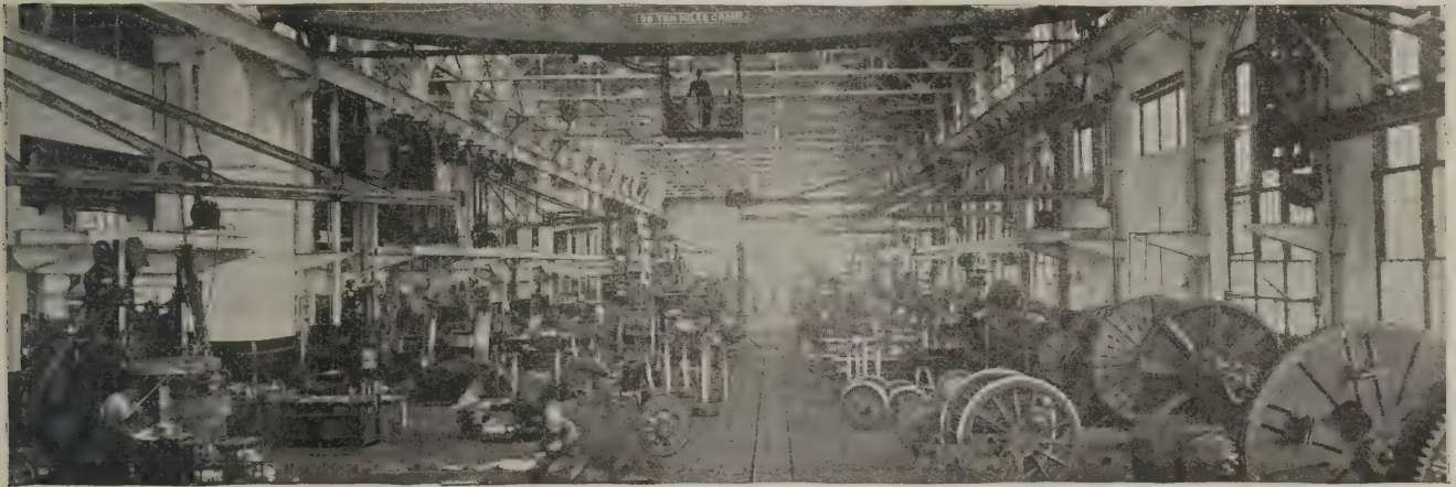
FIG. 3. GENERAL VIEW OF MACHINE SHOP, SHOWING ELECTRIC DRIVES.
